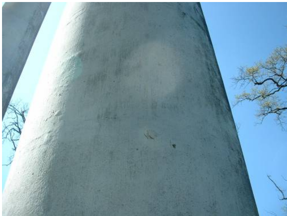
Photo 7 Overview of corrosion bursts of reinforcements behind the coating
