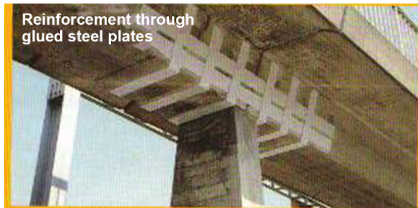
Figure 4.8. Bonding of metal plates (document by SIKa)
