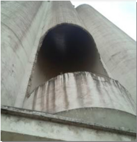
Figure 1.12. Opening of the skirt of the silo following the implementation of an internal lining
