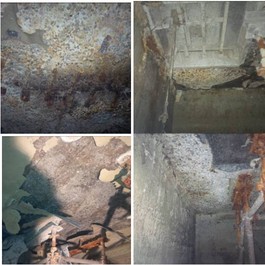
Figure 3.26. Examples of sulfate reactions on a mud tarpaulin (waste water plant)
