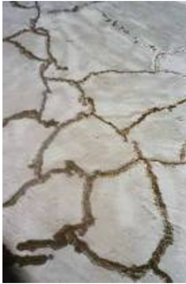
Figure 4.30. Injected cracks
