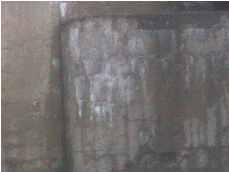
Figure 3.33. Alkali reaction in a retaining wall (St Hyacinthe-Quebec)
