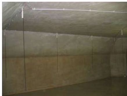
Figure 4.35. Tank cover dome after implementation of a cathodic protection
