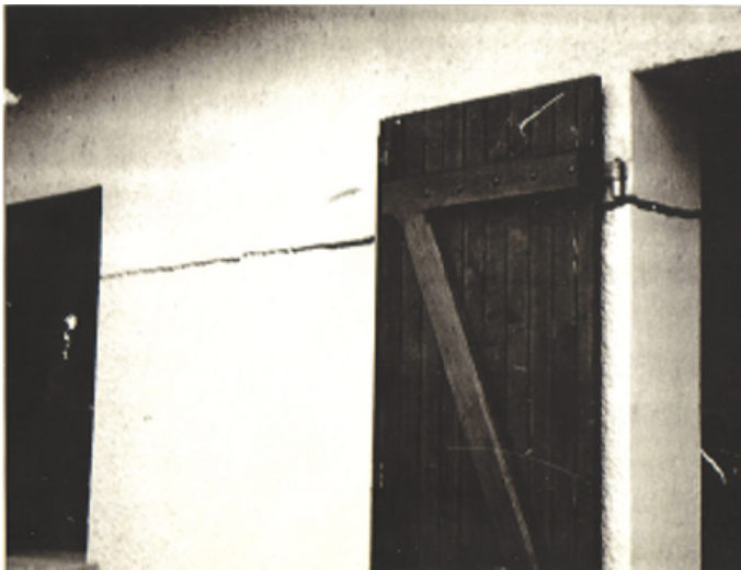
Figure 3.51. Cracking connected to the foundation mode on swelling soils
