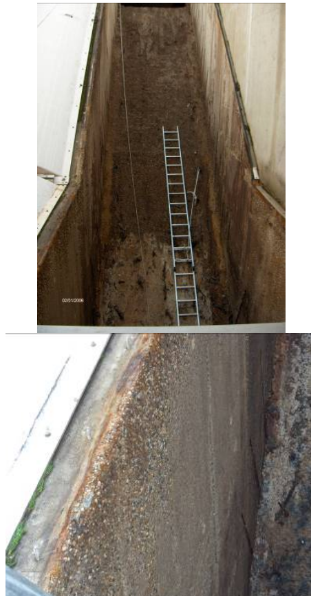
Figure 3.30. Example: sulfate attack at the foot of the lifting screws of a waste water plant
