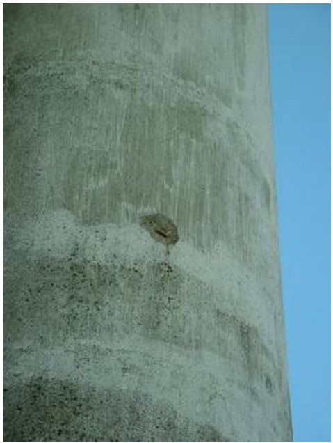
Photo 4 Beginning of corrosion of the reinforcements after carbonation of the concrete
