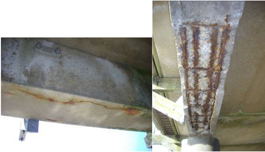
Figure 3.42. Example of marine salt attacks
