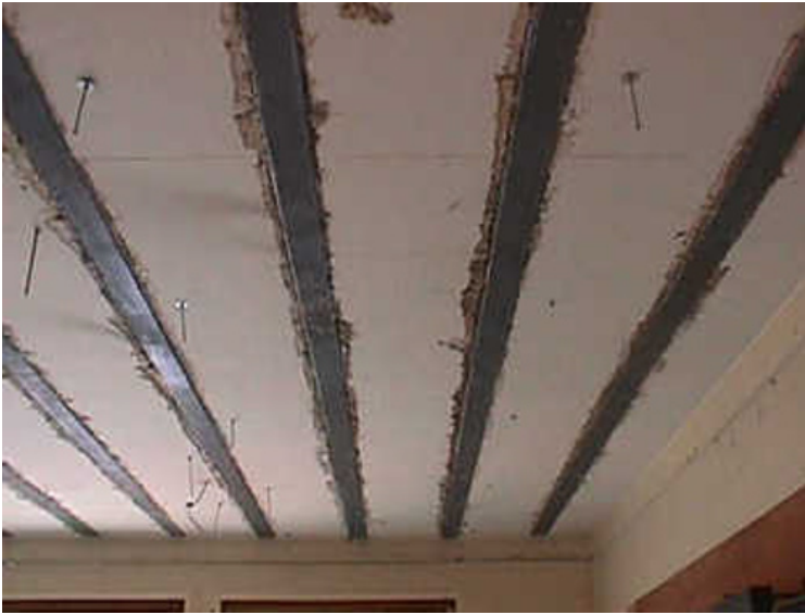
Figure 4.1. Example of floor reinforcement
