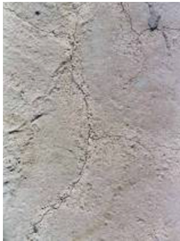
Figure 4.29. Shrinkage cracks before injection
