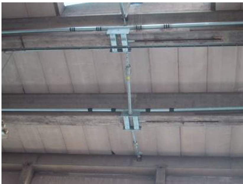
Figure 4.19. Example of beam reinforcement
