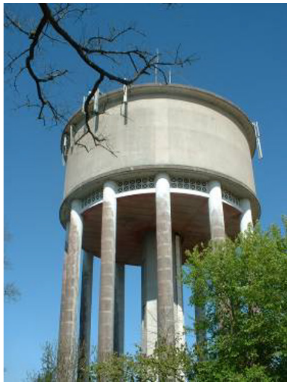
Photo 8 Deterioration of column paint
