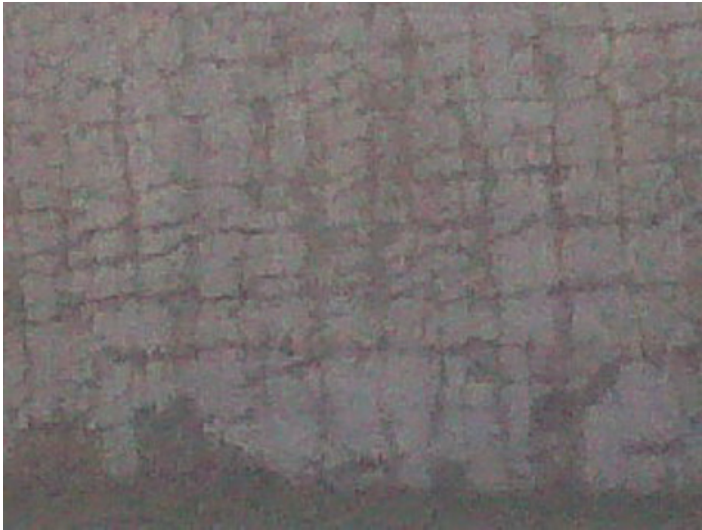
Figure 3.32. Concrete cracking (St Hyacinthe-Quebec retaining wall)
