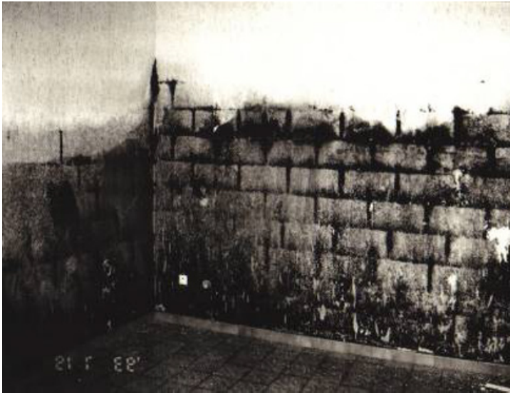
Figure 3.56. Lack of waterproofing in a buried construction
