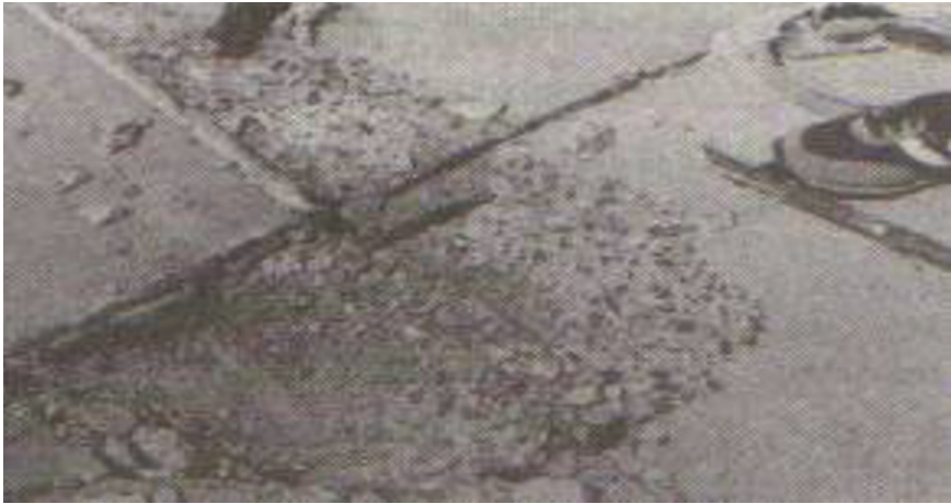
Figure 3.34. Burst cones for aggregates
