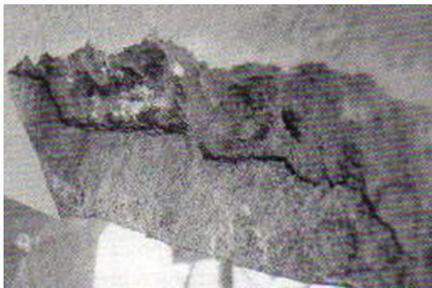
Figure 4.28. Failure of repair due to incorrect preparation of support
