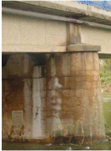
Figure 3.28. ISR on a river bridge pile
