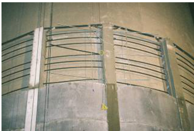
Figure 4.20. Silo reinforcement
