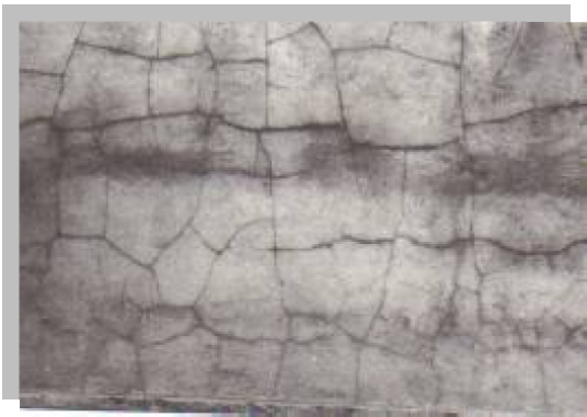
Figure 3.8. Example of cracking by plastic shrinkage
