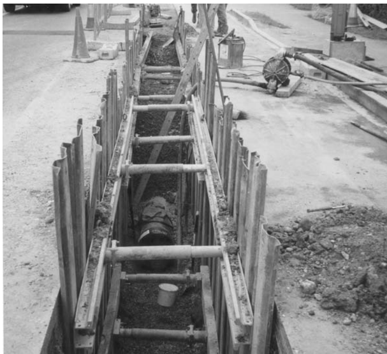
Plate 9b. A properly supported trench
