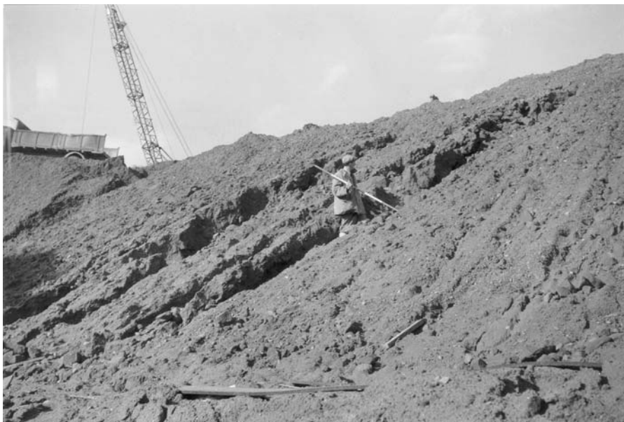
Plate 7a. Erosion of a newly placed embankment by rainfall runoff from the formation above. This is likely to be a contractor's risk, as it is 'a condition due to weather conditions' under ICE conditions Clause 12
