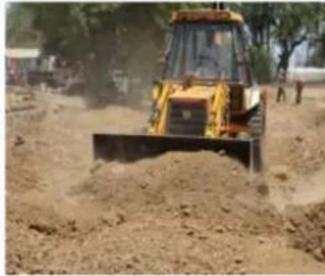
Preparation of ground
