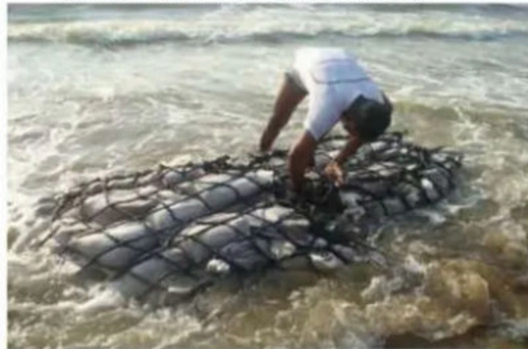
TYING OF ROPE GABIONS
