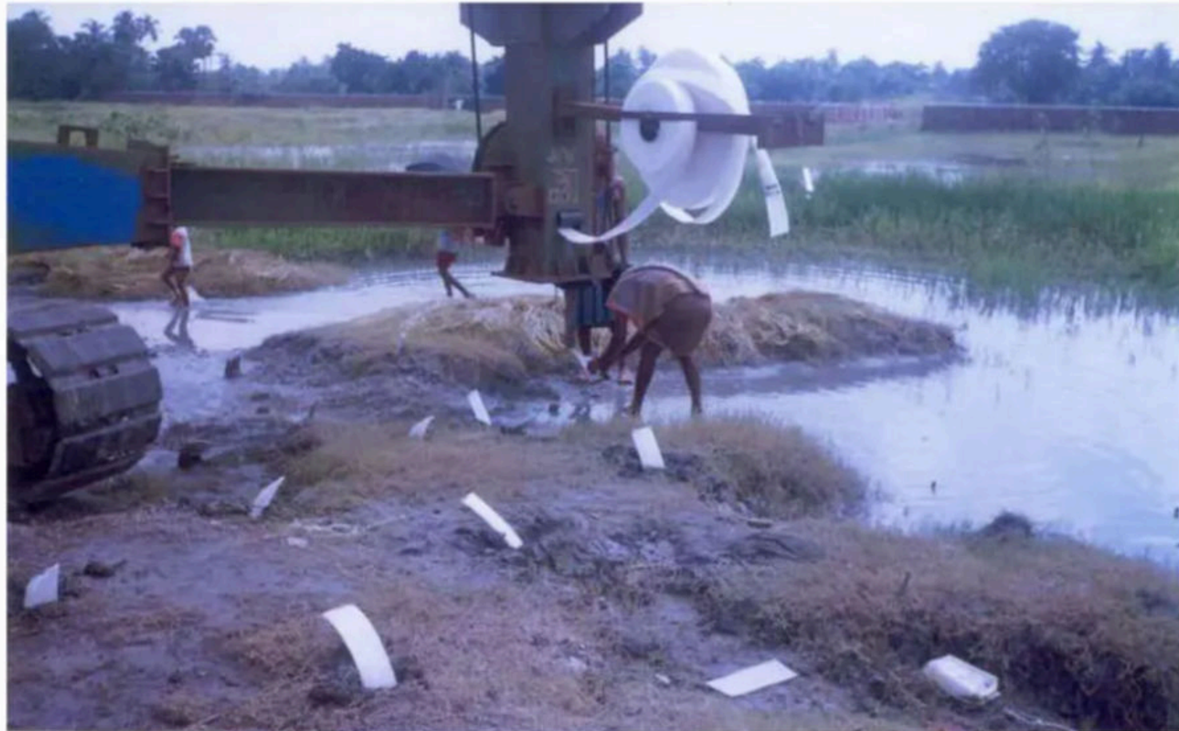
PVD being pushed into the ground
