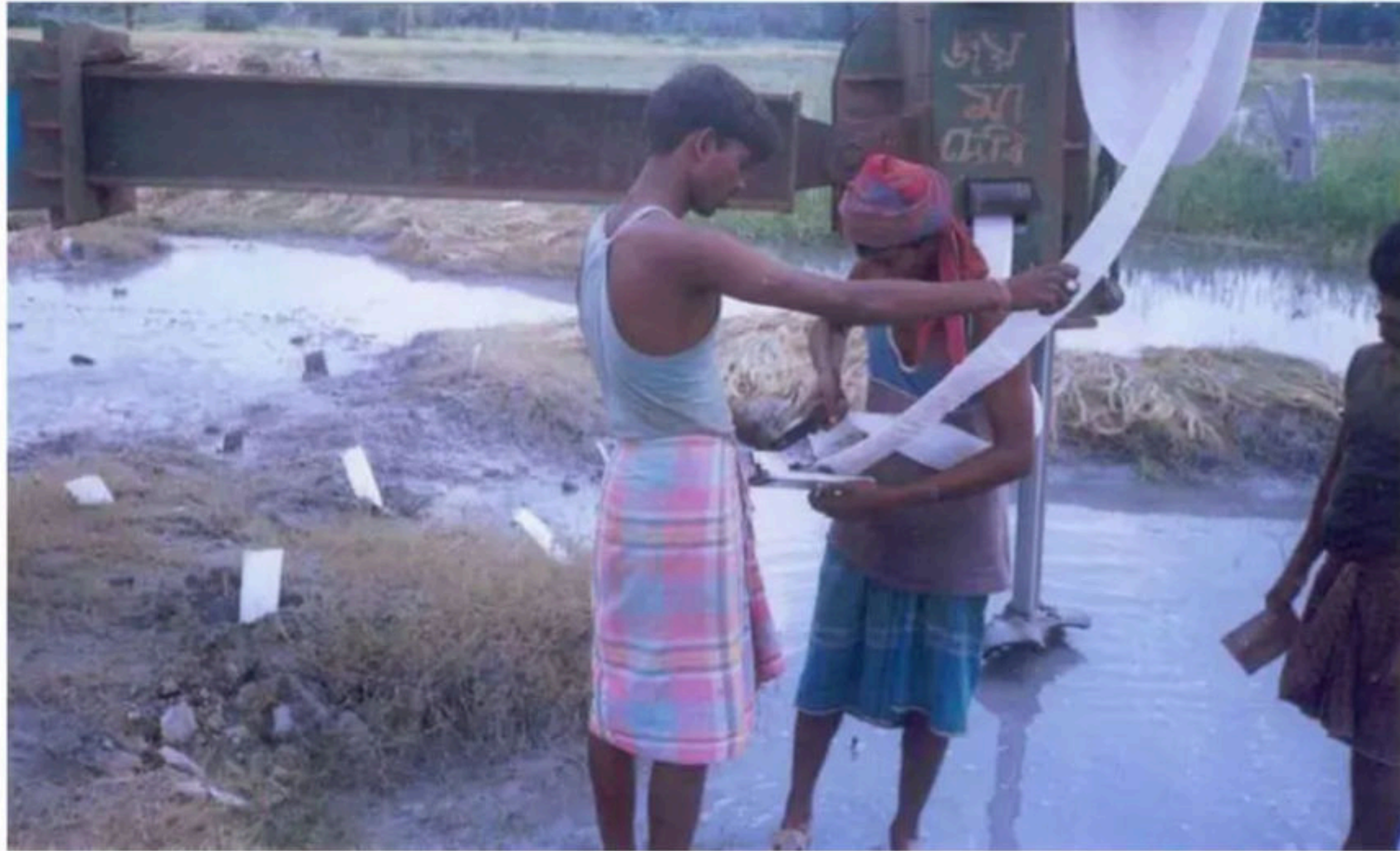
Installation of PVDs at a construction site – notice the connection of PVD with the anchor plate
