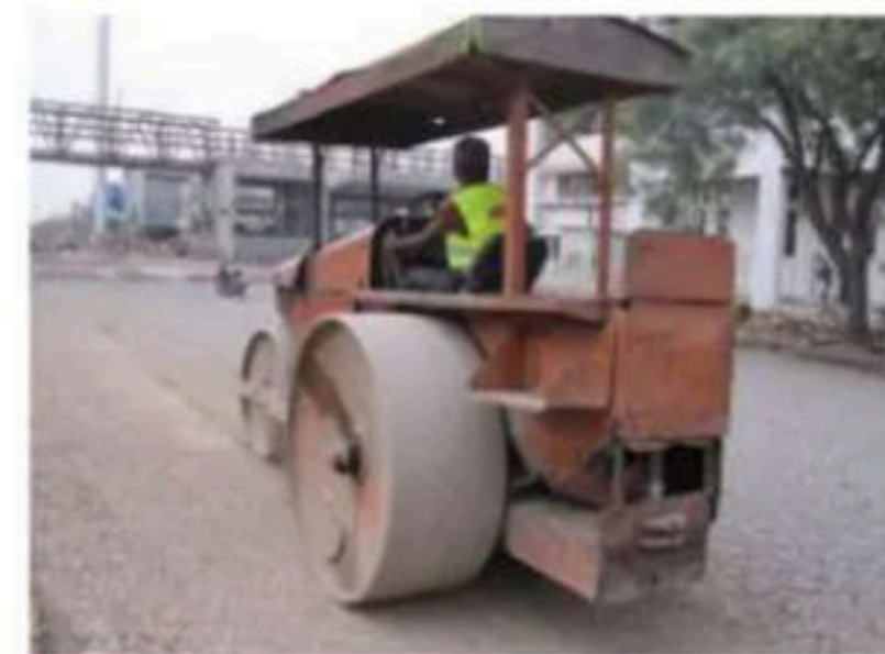
Compaction by a 10 tonne roller
