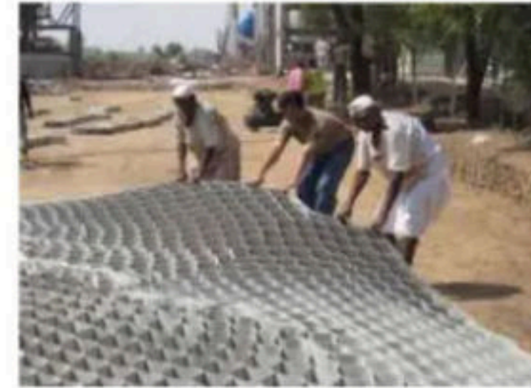
Stretching of the geocell layer
