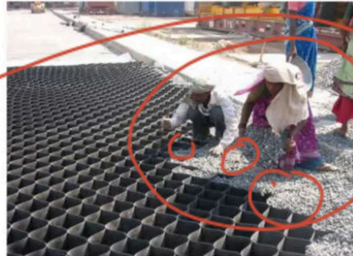
Geocell layer laid on the geotextile separator and filled with stone aggregate
