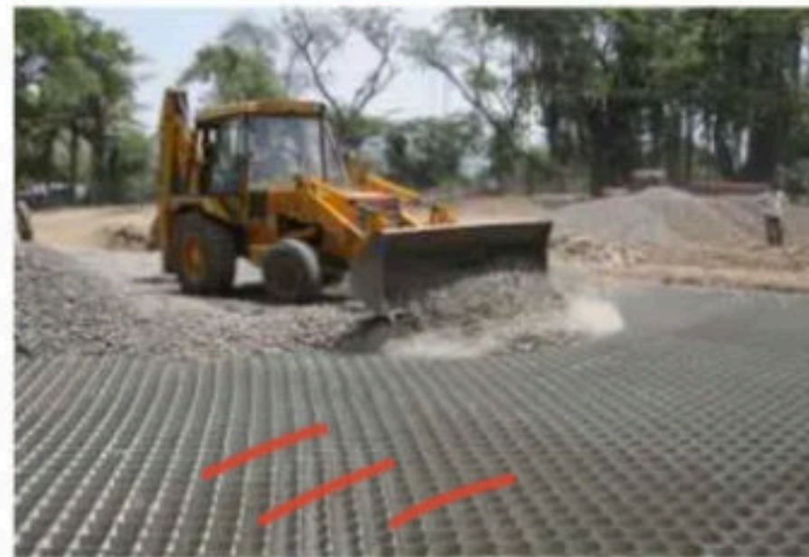
Stone aggregate filled in geocell pockets
