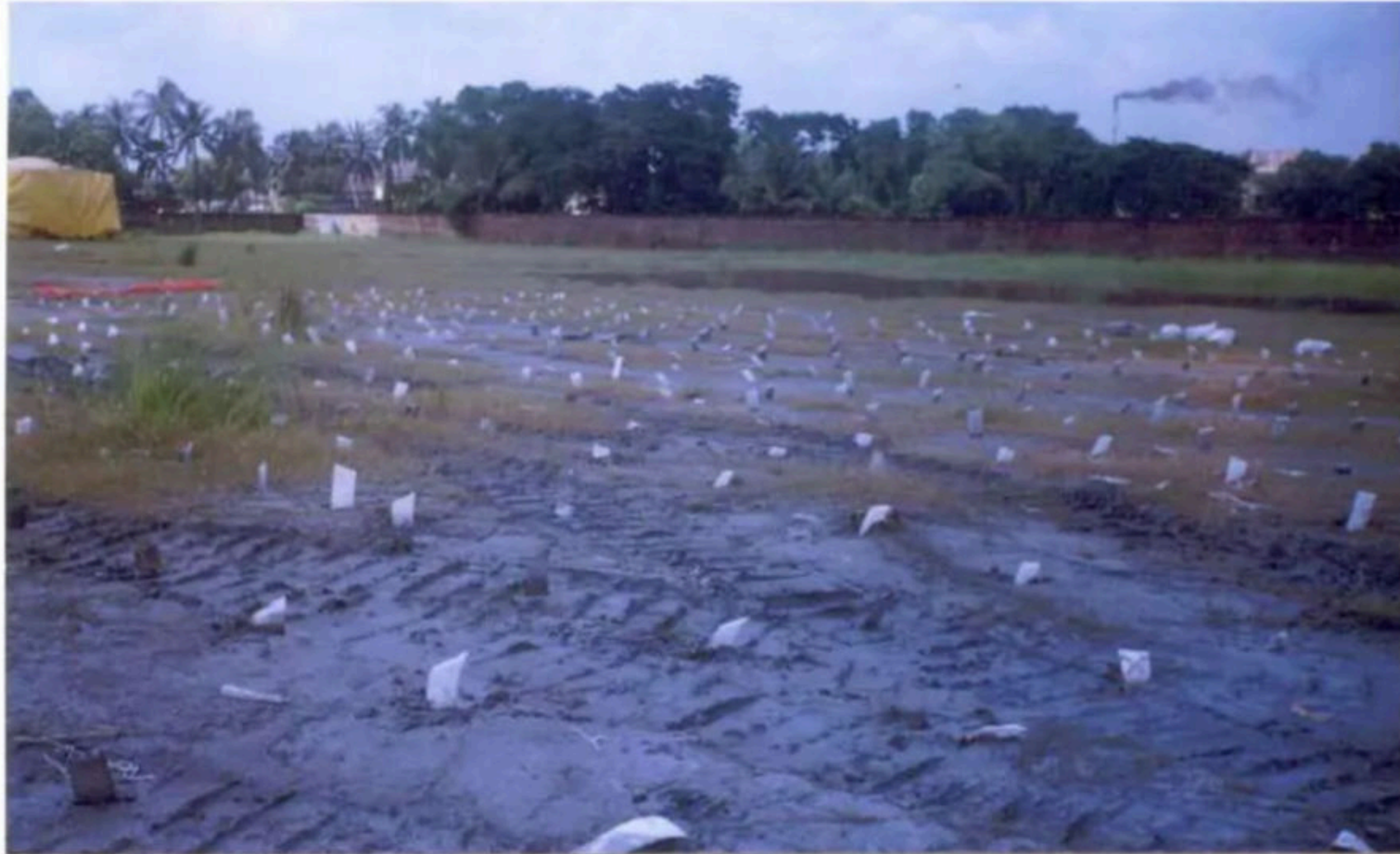
General view after installation of PVD' s at a site
