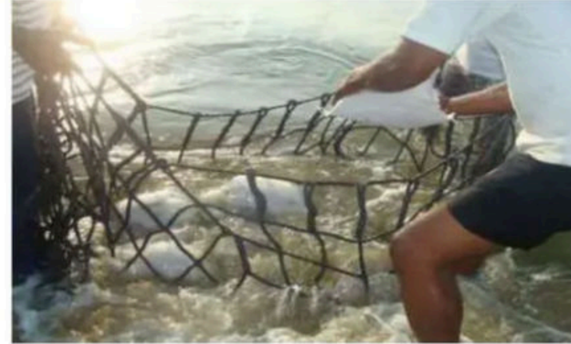
PLACEMENT OF GEOBAGS
