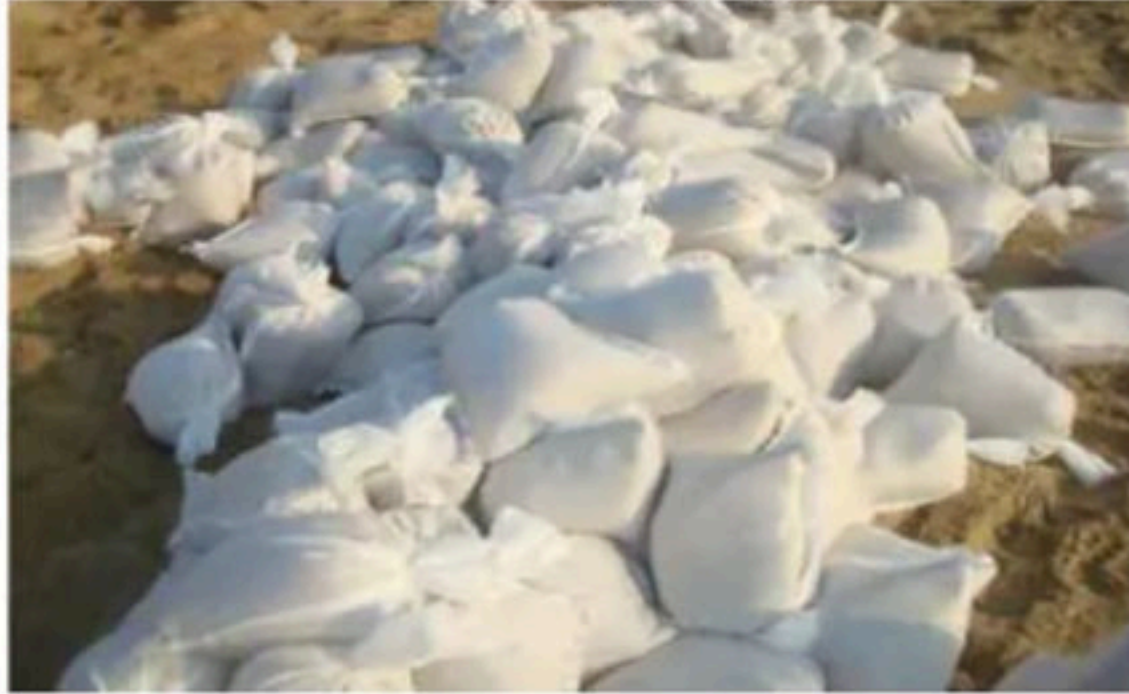
SAND FILLED GEOBAGS
