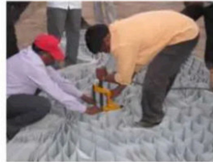
Stapling to join different geocells
