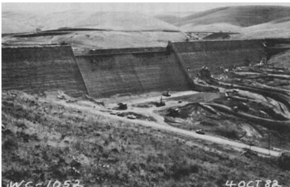
Figure 12-29 Willow Creek Dam, Oregon, the world's first all-roller-compacted concrete structure, shown about 18 weeks after the start of placement. (Photograph courtesy of Schrader, E., Concr. Int. , Vol. 6, No. 5, 1984.)
