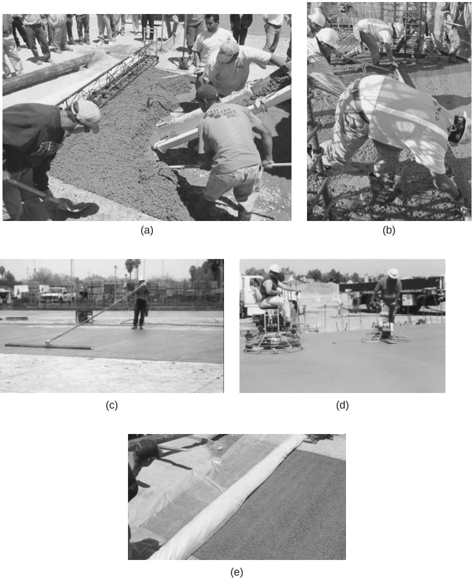
Figure 10-4 Placement and finishing of concrete slabs.
