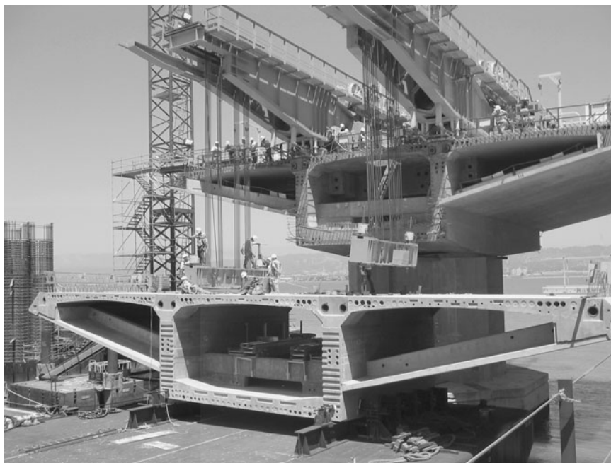
Figure 1-9 Precast concrete girders under installation for the Skyway Segment of the eastern span crossing the San Francisco Bay. (Photograph courtesy of Joseph A. Blum.)
