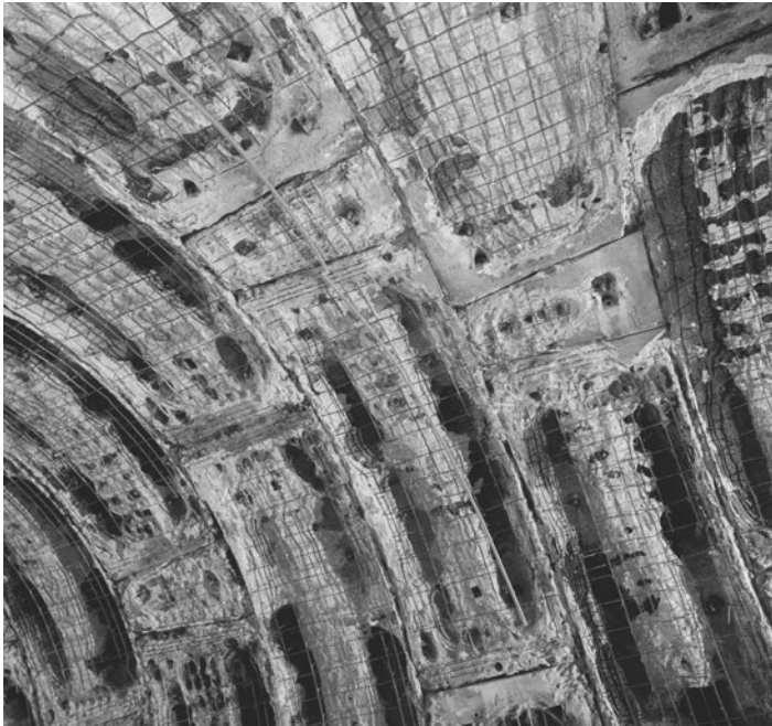
Figure 5-13 Fire damage to the concrete lining of the Channel Tunnel. [Photograph courtesy of Paul Acker]
