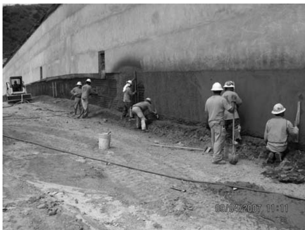
FIGURE 2.2 Shortcrete lagging. (Illustration provided by Malcolm Drilling.)
