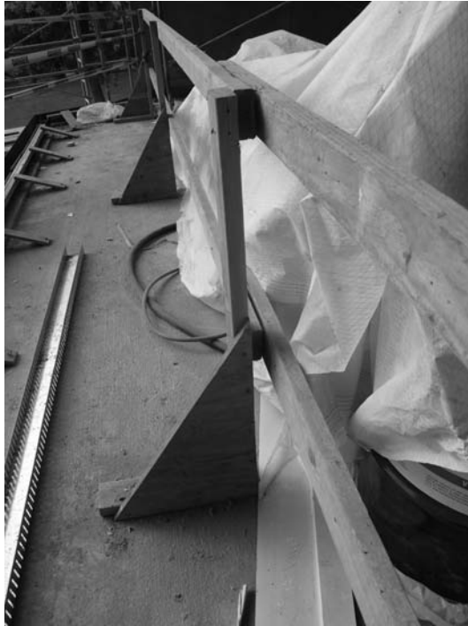
FIGURE 48.2 Wood guardrails. (Photo by author, courtesy of Hathaway Dinwiddie Construction Company and California State University Northridge.)
