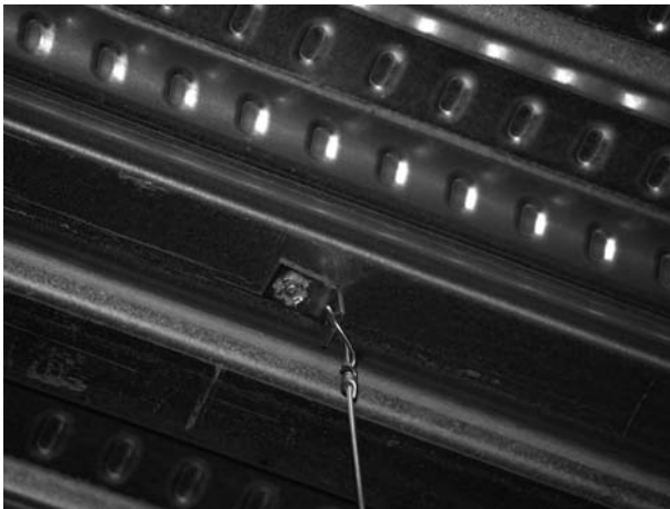
FIGURE 32.2 Acoustical ceiling wire hung with shot pin. (Photo by author, courtesy of Hathaway Dinwiddie Construction Company and The California Institute of Technology.)
