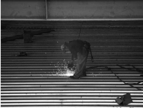
FIGURE 11.2 Shooting studs. (Photo by author, courtesy of Hathaway Dinwiddie Construction Company and Tishman Speyer.)
