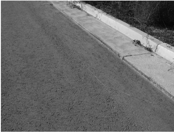
FIGURE 43.1 Initial AC paving lift for construction purposes. (Photo by author, courtesy of Hathaway Dinwiddie Construction Company and Tishman Speyer.)
