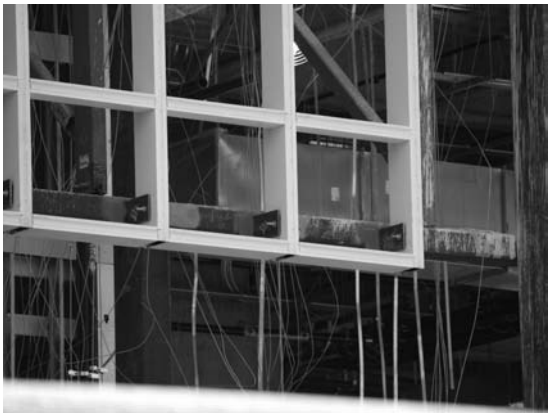
FIGURE 22.6 Curtain wall base support.
