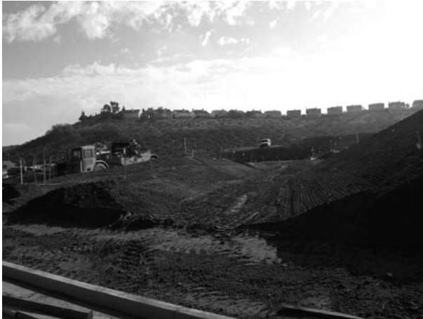
FIGURE 3.6 Site grading. (Photo by author, courtesy of Hathaway Dinwiddie Construction Company and Tishman Speyer.)
