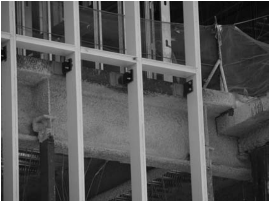
FIGURE 22.5 Curtain wall intermediate support.
