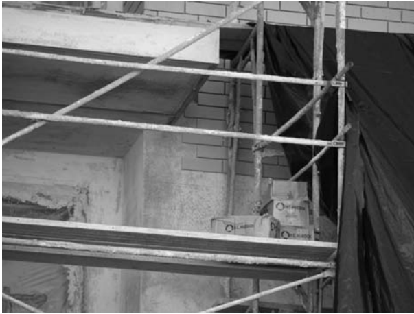
FIGURE 16.2 Thin brick on top of plaster base.
