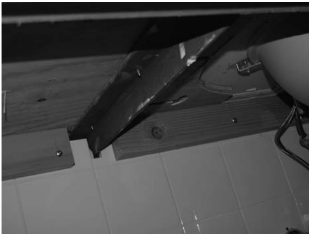
FIGURE 12.8 Counter support angles. (Photo by author, courtesy of Hathaway Dinwiddie Construction Company and The California Institute of Technology.)
