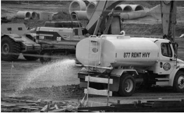
FIGURE 3.5 Dust control. (Photo by author, courtesy of Hathaway Dinwiddie Construction Company and Tishman Speyer.)
