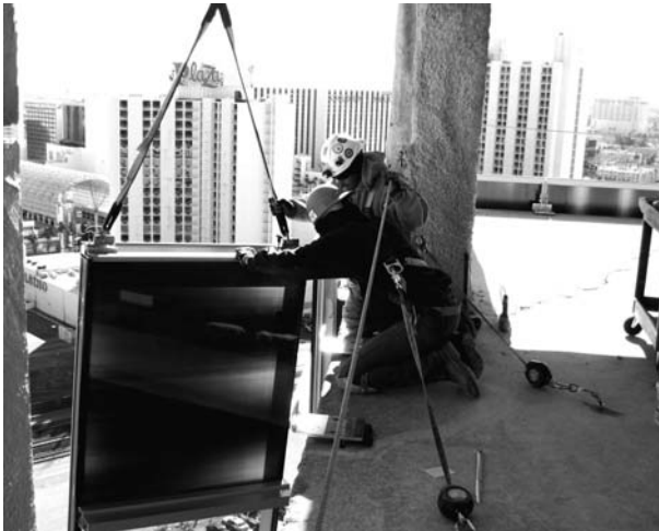
FIGURE 22.2 Curtain wall installation. (Photo provided by Walters and Wolf, Inc.)
