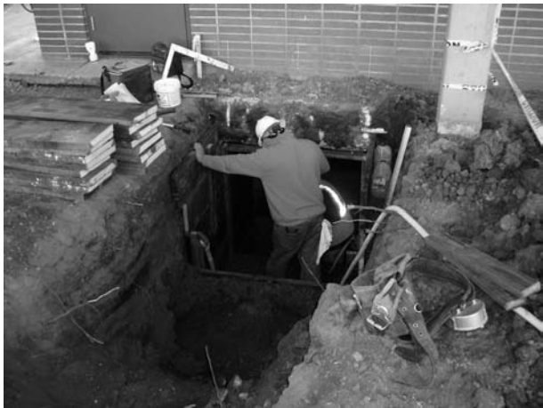
FIGURE 2.11 Underpinning. (Illustration provided by Malcolm Drilling.)
