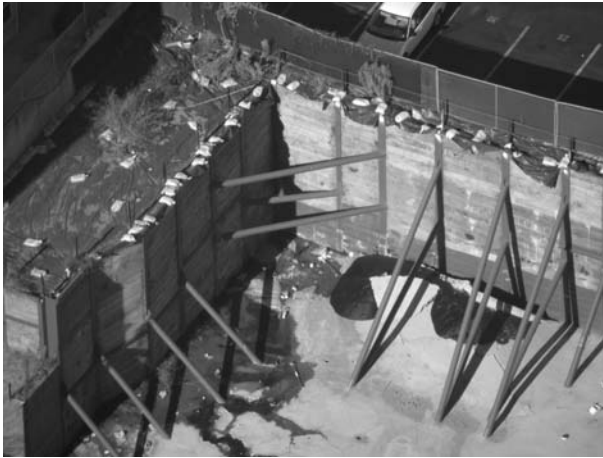
FIGURE 2.12 Rakers and corner bracing.
