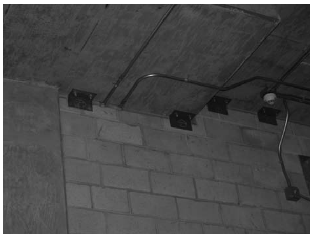
FIGURE 12.3 CMU wall clips. (Photo by author, courtesy of The University of Southern California.)
