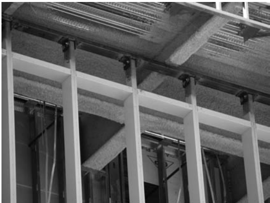
FIGURE 22.4 Curtain wall head support.
