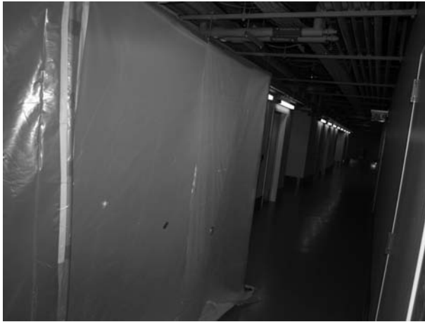
FIGURE 1.2 Dust barrier to isolate construction work area from occupied spaces on renovation projects. (Photo by author, courtesy of Hathaway Dinwiddie Construction Company and California Institute of Technology.)
