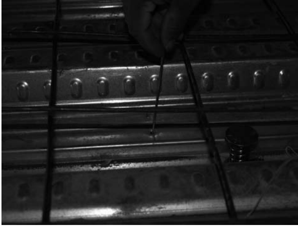
FIGURE 32.1 Dropping ceiling wires through metal decking. (Photo by author, courtesy of Hathaway Dinwiddie Construction Company and Tishman Speyer.)
