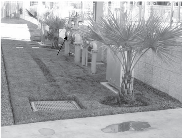
FIGURE 38.2 Backflow preventer.
