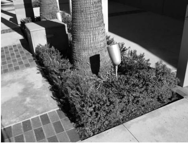
FIGURE 44.2 Large trees must at times be set ahead of the concrete paving the root ball for this tree is wider than the opening in the sidewalk. (Photo by author, courtesy of The University of Southern California.)
