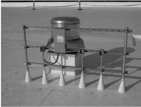
FIGURE 47.7 Roof jack spacing. (Photo by author, courtesy of Hathaway Dinwiddie Construction Company and The California Institute of Technology.)
