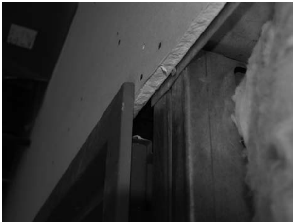
FIGURE 26.1 Door frame. (Photo by author, courtesy of Hathaway Dinwiddie Construction Company and California State University Northridge.)
