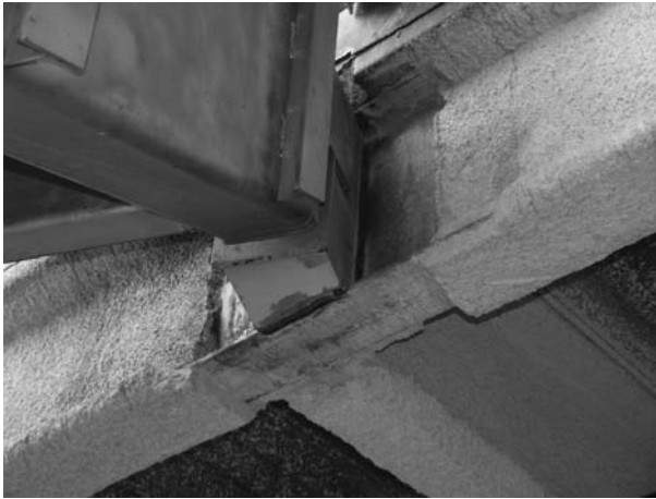
FIGURE 14.2 Scraped fireproofing.
