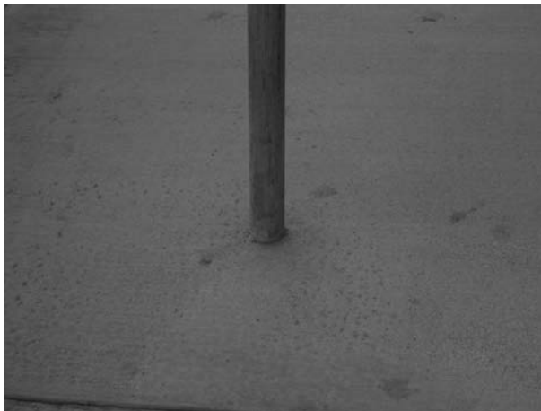
FIGURE 45.1 Post set ahead of concrete paving. (Photo by author, courtesy of The University of Southern California.)
