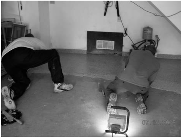
FIGURE 31.1 Epoxy flooring application. (Photo provided by Hi-Tech Flooring.)
