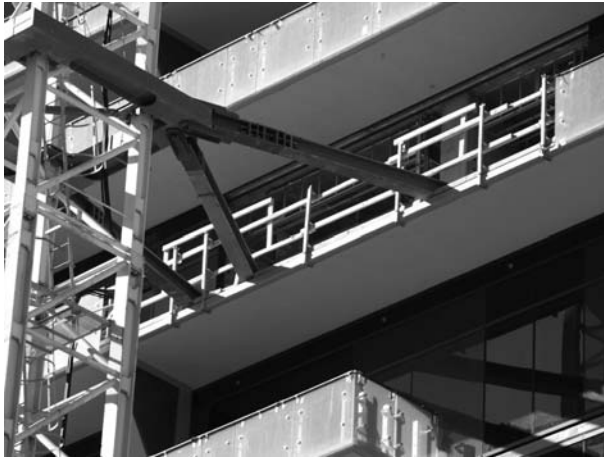
FIGURE 47.2 Tower crane lateral support at building deck.
