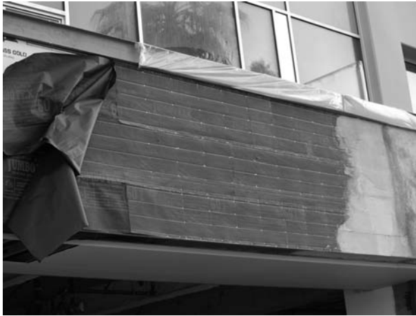
FIGURE 16.1 Plaster installation.
