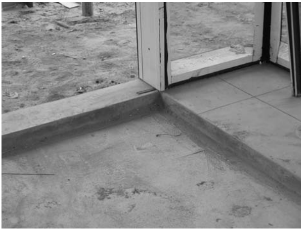
FIGURE 35.13 Blockout for a recessed floor mat. (Photo by author, courtesy of Hathaway Dinwiddie Construction Company and The California Institute of Technology.)
