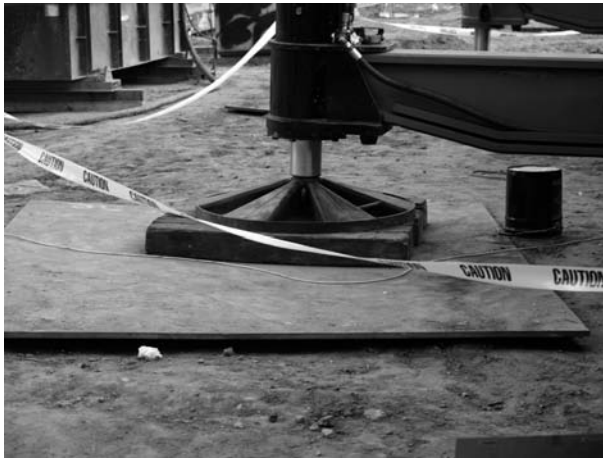
FIGURE 47.5 Trench plate dispersing load of crane outrigger. (Photo by author, courtesy of Hathaway Dinwiddie Construction Company and Tishman Speyer.)
