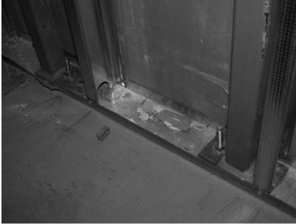
FIGURE 12.7 Low wall posts. (Photo by author, courtesy of Hathaway Dinwiddie Construction Company and The California Institute of Technology.)
