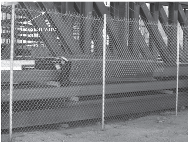
FIGURE 45.3 Chain link fence with tension wire.
