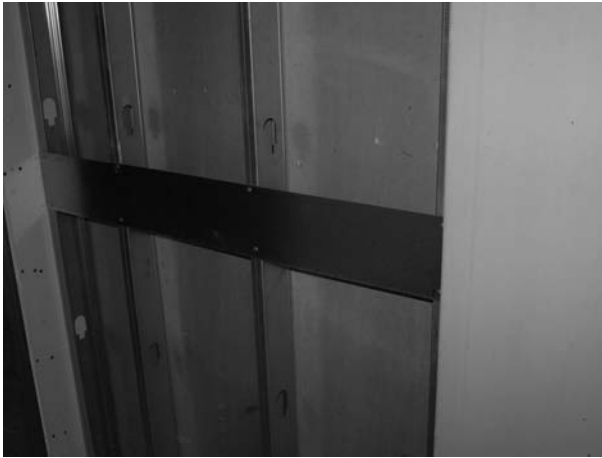
FIGURE 24.2 In-wall backing. (Photo by author, courtesy of Hathaway Dinwiddie Construction Company and The California Institute of Technology.)
