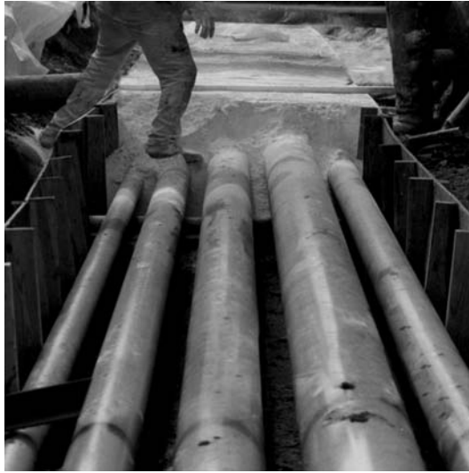
FIGURE 42.3 DriTherm insulation. (Photo provided by DriTherm International.)
