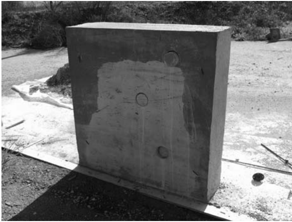
FIGURE 9.1 Shotcrete test panel. (Photo by author, courtesy of Hathaway Dinwiddie Construction Company and Tishman Speyer.)
