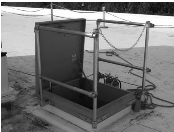
FIGURE 35.9 Roof hatch. (Photo by author, courtesy of Hathaway Dinwiddie Construction Company and The California Institute of Technology.)
