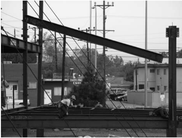
FIGURE 10.1 Steel erection. (Photo by author courtesy of Hathaway Dinwiddie Construction Company and Tishman Speyer.)
