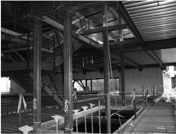
FIGURE 10.4 Elevator steel. (Photo by author, courtesy of Hathaway Dinwiddie Construction Company and Tishman Speyer.)
