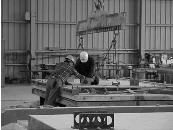
FIGURE 17.3 Precast concrete plant. (Photo provided by Walters and Wolf, Inc.)
