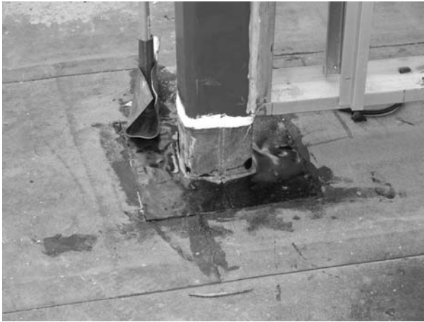
FIGURE 20.2 Lead roof jack. (Photo by author, courtesy of Hathaway Dinwiddie Construction Company and California State University Northridge.)
