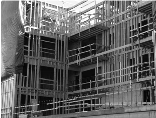
FIGURE 24.1 Stud framing.
