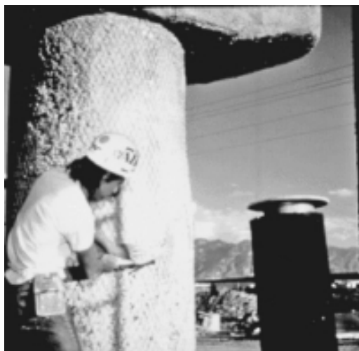
FIGURE 9.10 Fixing titanium on a concrete column.
