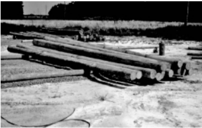
FIGURE 13.10 Preparation of wood piles.
