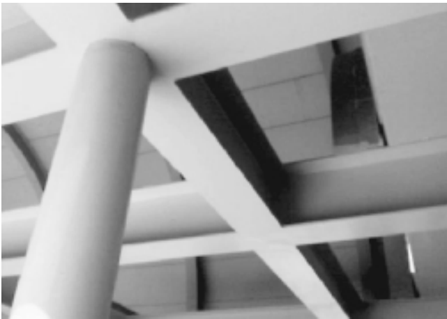
FIGURE 7.4 Photo of roof system.
