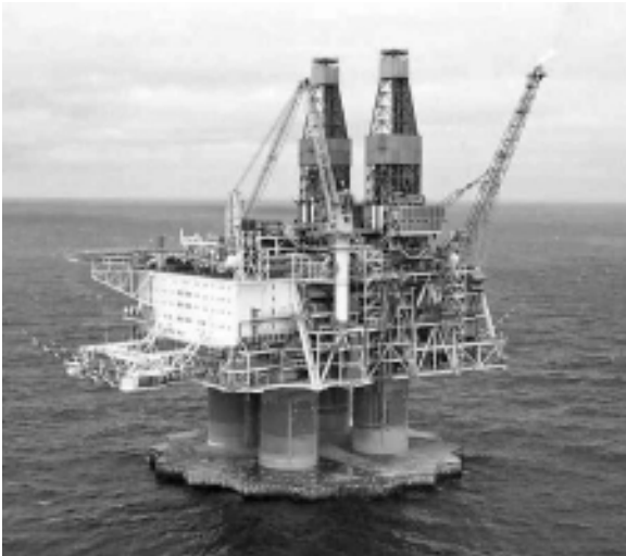
FIGURE 12.4 Concrete gravity platform.
