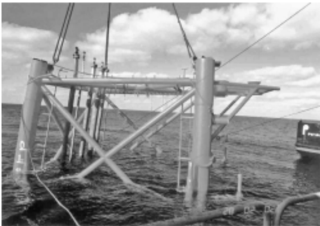
FIGURE 12.39 Lifting and installing of jacket.
