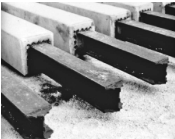
FIGURE 13.16 Composite section piles.
