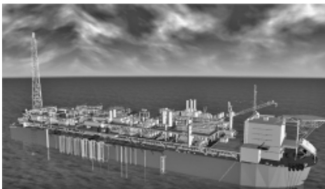
FIGURE 12.5 Floating production, storage, and offloading.
