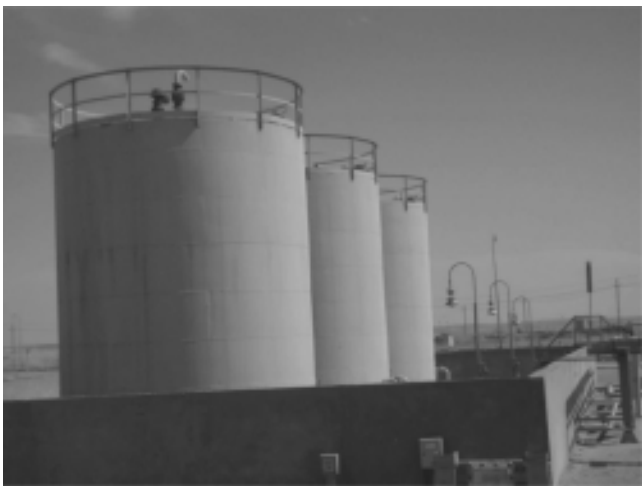
FIGURE 5.16 Condensate tanks inside a dike from retaining the wall.
