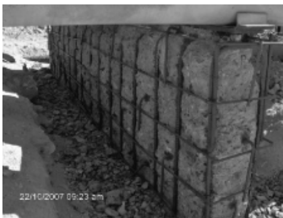
FIGURE 10.4 Repair of concrete pedestal.
