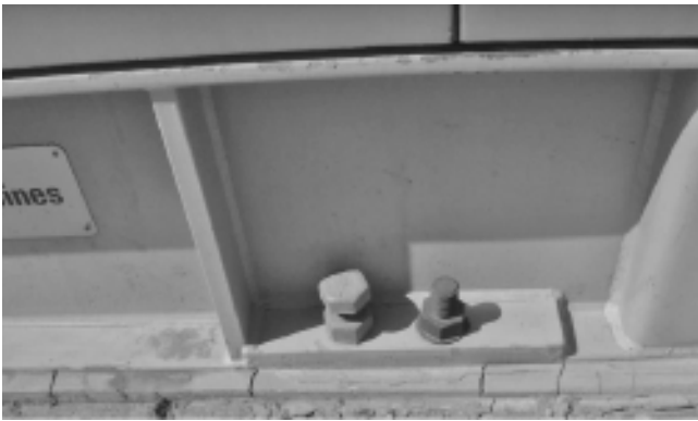
FIGURE 4.3 Fixing the skid to concrete.
