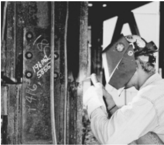
FIGURE 7.24 Welding in an existing building.
