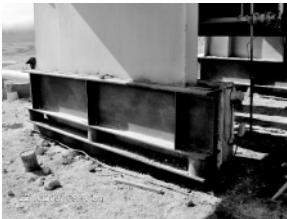
FIGURE 10.1 Temporary repair using steel sections.
