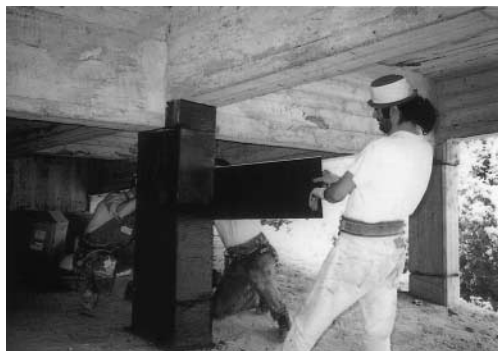
FIGURE 39.5 The use of REPLARK to wrap a column with carbon fibre polymer composite (photograph by kind permission of Sumitomo Corporation (UK) London).
