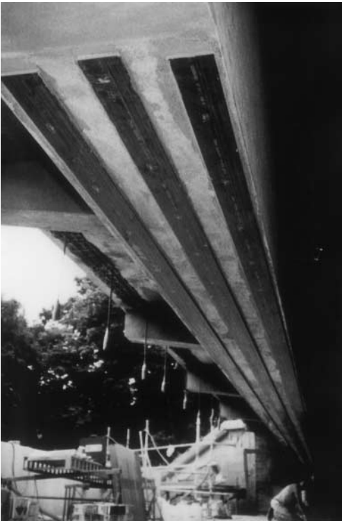
FIGURE 39.4 Plate bonding on the soffit of a bridge (photograph by kind permission of Sika Ltd, Welwyn Garden City, Herts, UK).
