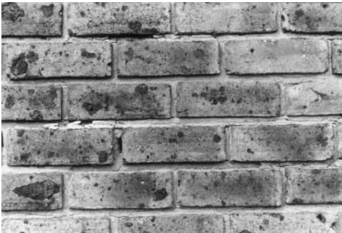
FIGURE 33.1 Sulfate attack.
