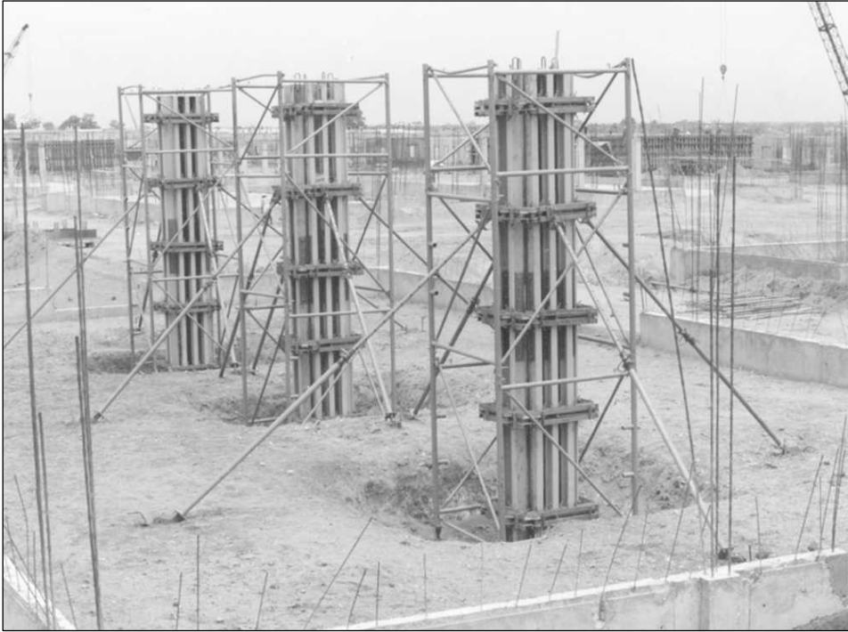
Figure 6.6 Application of L&T Column Formwork for the Construction of Factory.
