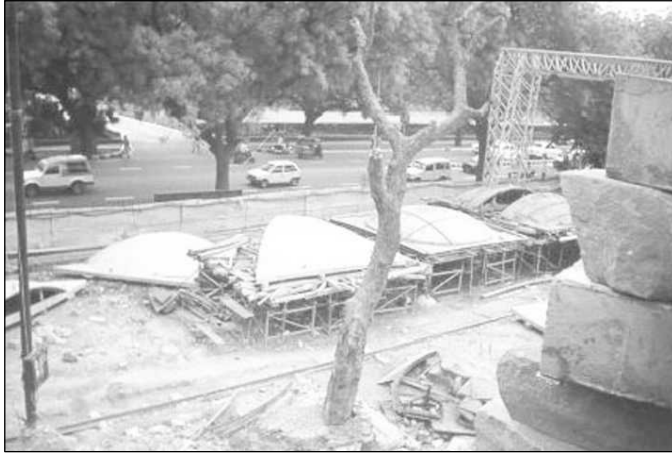
Figure 14.26 Another View of Casting of Bubbles for the Parliament Library Project.
