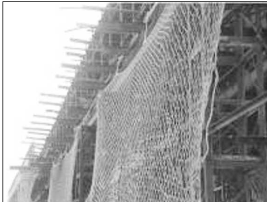
Figure 17.26 Safety Net not Properly Installed.
