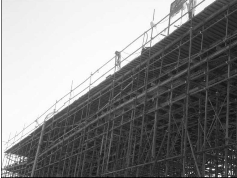
Figure 9.26 Arrangement of Tubular Steel Scaffolds for Casting Bridge Deck.
