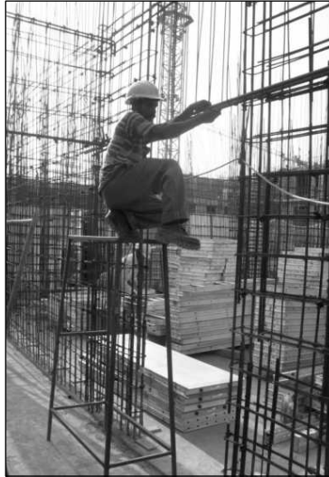
Figure 7.31 Vertical Rebar Fixing.
