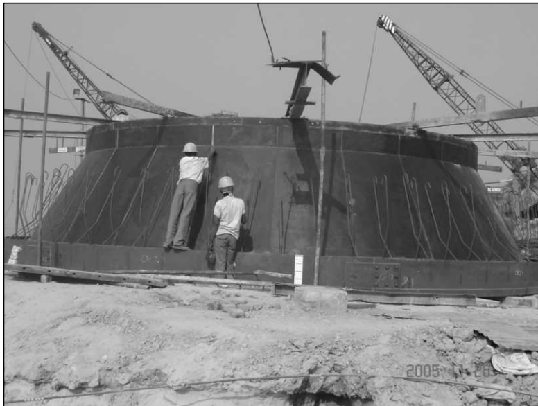
Figure 9.3 View Showing Inside Shutter in Position.
