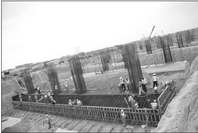
Figure 4.3 Formwork Arrangement for a Large Combined Footing Used at Delhi International Airport.
