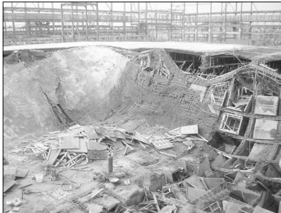
Figure 17.2 View of Collapsed Waffle Slab Segment.
