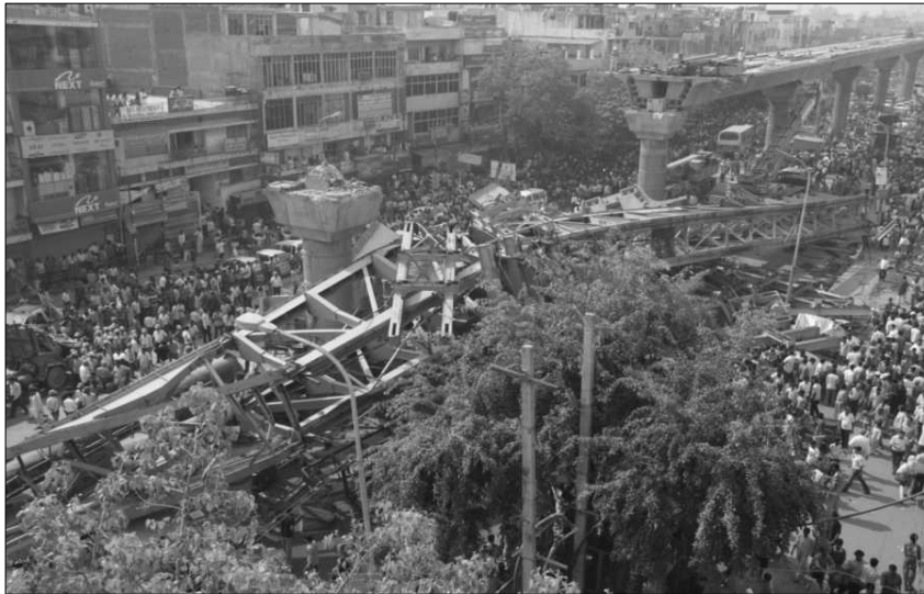
Figure 9.47 Collapse of Launching Girder in Laxmi Nagar.
