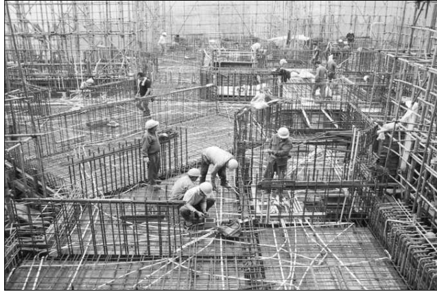
Figure 7.39 Deck Rebar and Second M&E Works in Progress.
