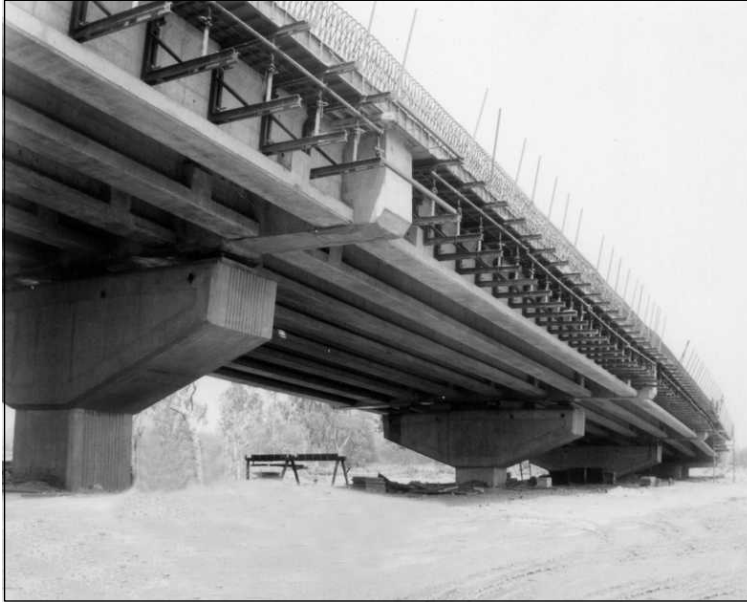
Figure 9.42 Formwork Arrangement (Accessible from Both Sides) of Parapets for Flyover in Delhi.
