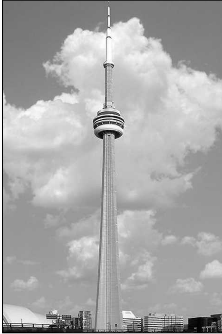
Figure 11.1 CN Tower at Toronto (One of the Early Slipformed Structures).
