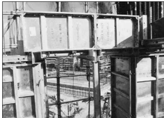
Figure 7.36 Beam Erection.
