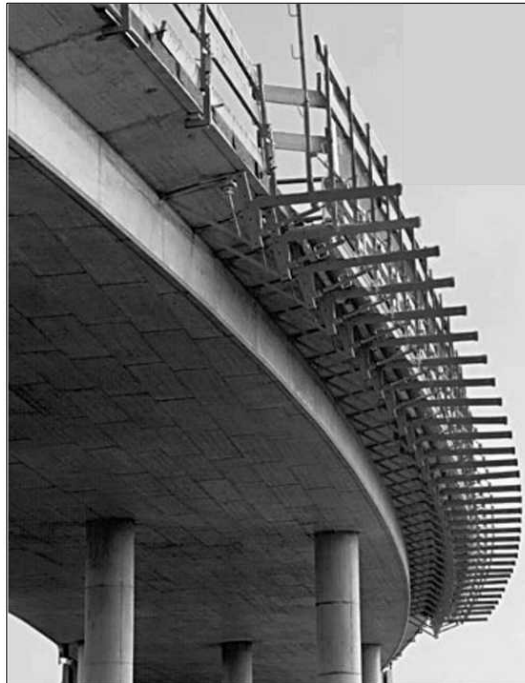
Figure 9.46 Field Application of Doka Edge Beam Formwork Solution.
