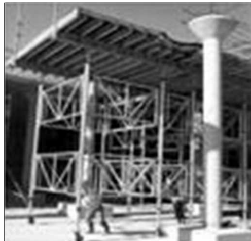
Figure 10.4 Harsco Infrastructure Flying Table Form Being Assembled.
