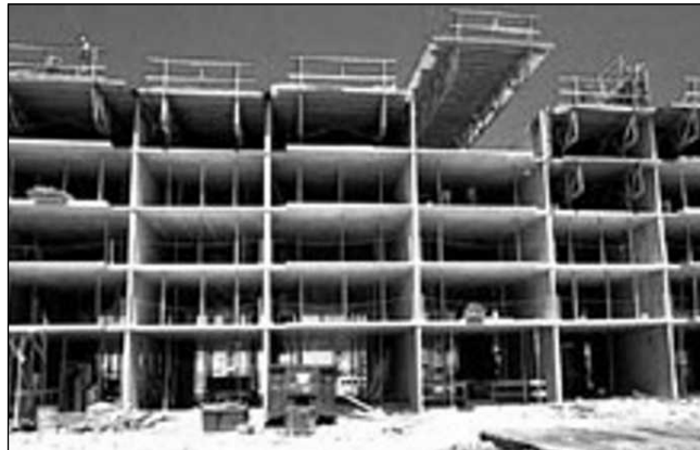
Figure 10.2 Interform Aluminium Flying Forming System in Use.
