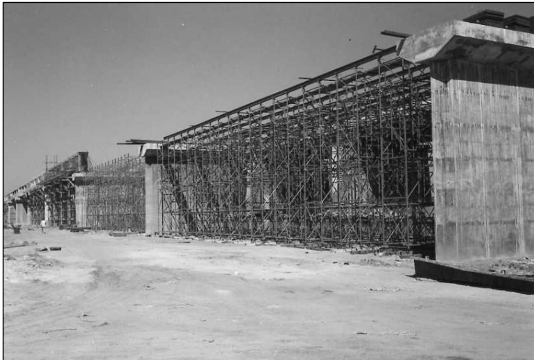
Figure 9.27 L&T Heavy Duty Tower System in Use for Deck Slab and Girder Formwork Support.
