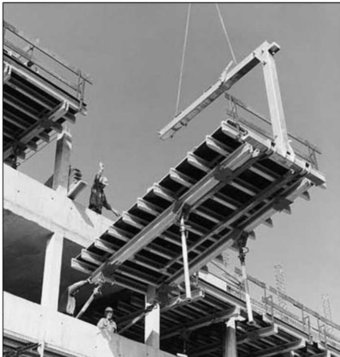
Figure 10.19 Table Module Being Shifted to New Location (Note the Props in Folded Position) (Courtesy PERI).
