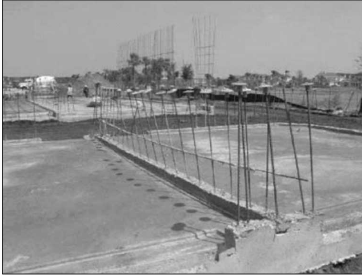
Figure 10.27 Construction of Starter Wall for the Tunnel Formwork System.
