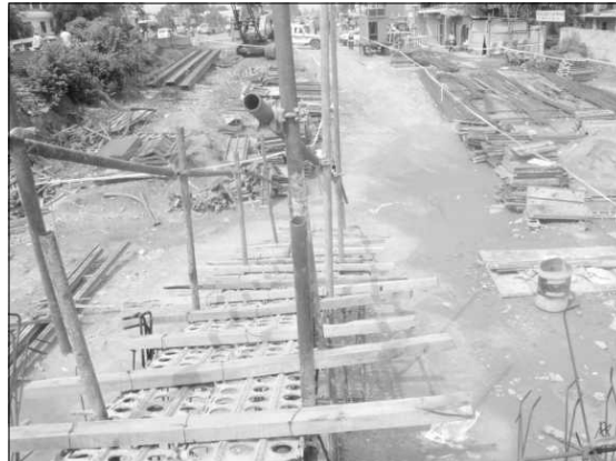
Figure 17.20 Another Type of Makeshift Ramp.
