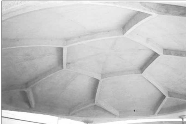
Figure 14.27 Rib Pattern on the Inner Surface of Bubbles for the Parliament Library Project.
