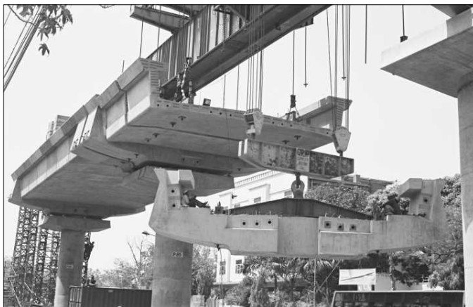
Figure 14.40 Pier Segment Being Raised (Note Lifting Tackle, Weight 75 ton).
