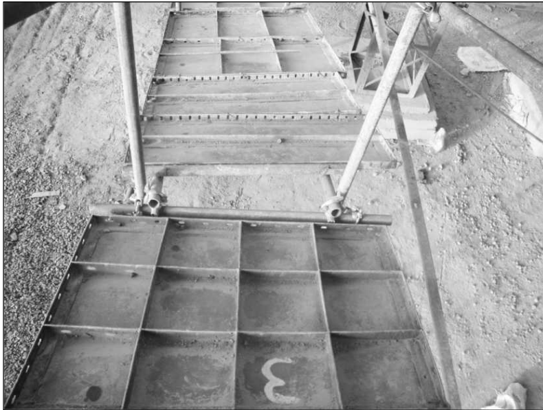
Figure 17.28 Makeshift Ramp Along with Dangerous Gaps (Openings) in between.
