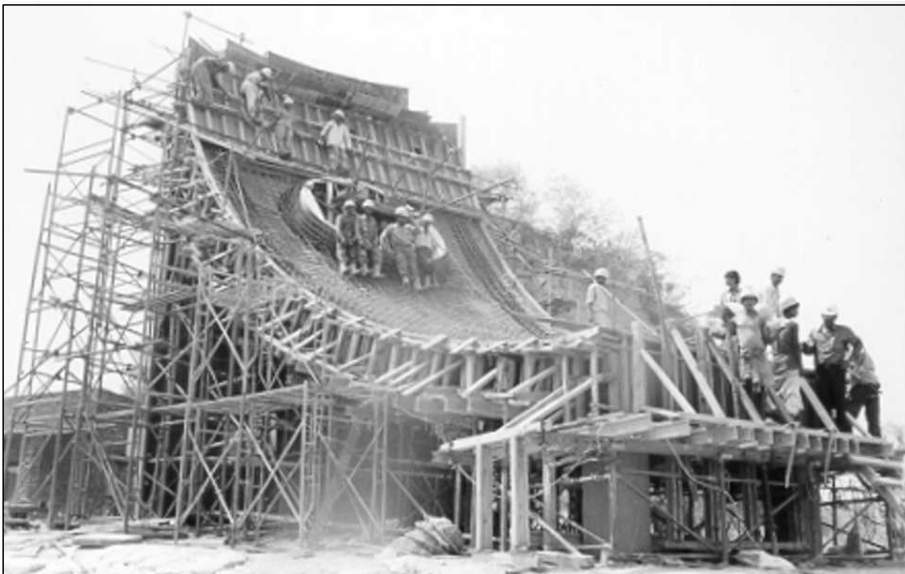
Figure 16.8 Mock Up of Sloping Roof in Progress.
