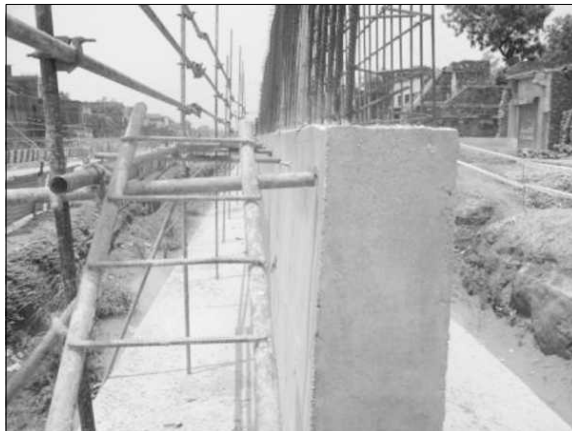
Figure 17.24 Ladder Resting on Pipes which in Turn is Supported on Reinforcement Inserted into Weepholes of the Concrete Wall.
