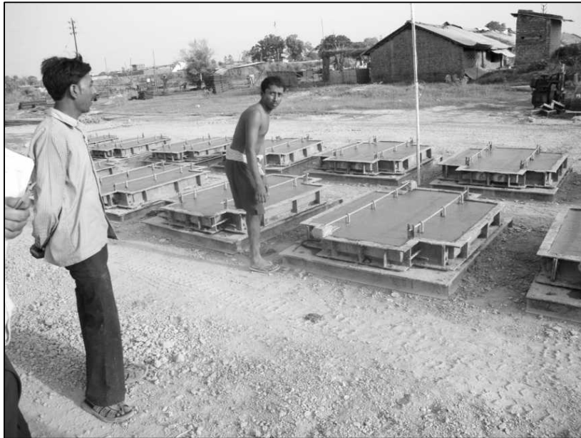
Figure 14.4 Steel Moulds in Use for Casting Wall Panels for an Underpass.
