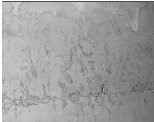
(e) Plywood Grains Stuck on the Concrete Surface
