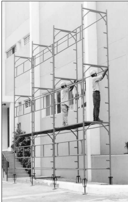
Figure 13.13 Scaffolds Primarily for Access (Courtesy L&T Formwork).
