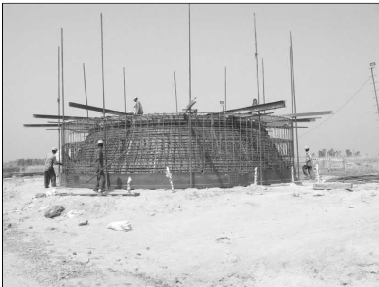
Figure 9.4 View Showing Reinforcement in Position.
