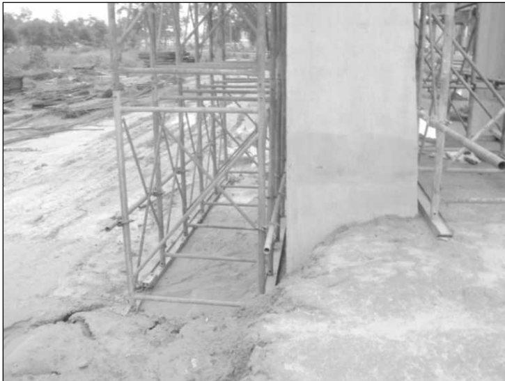
Figure 17.41 Erosion of Soil Beneath the Shoring Was Noticed.
