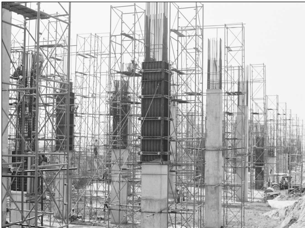
Figure 6.28 Column Construction Using Steel Formwork for Delhi International Airport Project.
