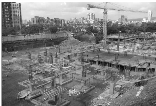
Figure 10.17 Extensive Use of Tableform at Oberoi Mall Project Site Mumbai (Courtesy L&T Formwork).
