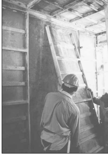
Figure 7.41 Striking of Wall Formwork.
