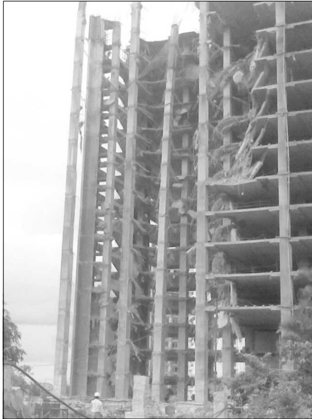
Figure 17.1 Collapse of One Floor Leading to Another.
