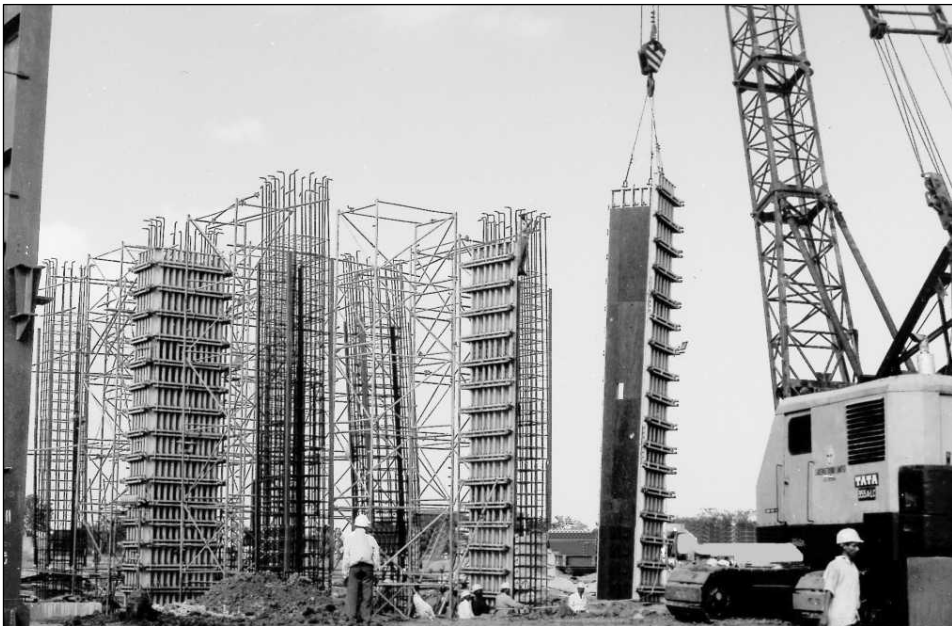
Figure 6.7 Column Formwork Being Lifted With the Help of a Crane.
