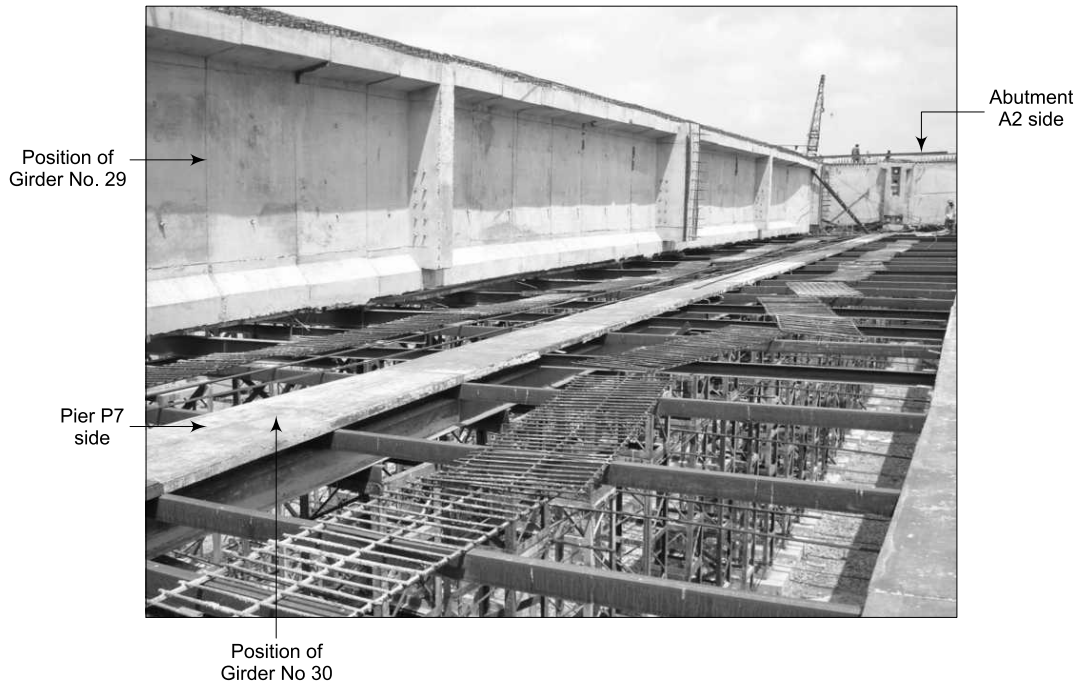
Figure 9.51 View of Dislocated Shutters.
