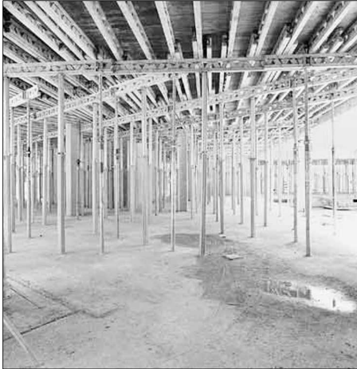
Figure 7.25 Multiflex Girder Slab Formwork (All Components in Position) (Courtesy PERI).
