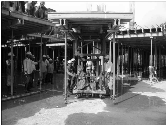
Figure 10.15 Table Formwork Being Positioned (Courtesy L&T Formwork).
