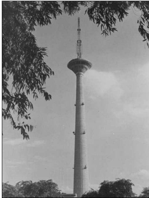
Figure 11.2 Pitampura TV Tower in New Delhi, 235 m Height Constructed Using Slipform.
