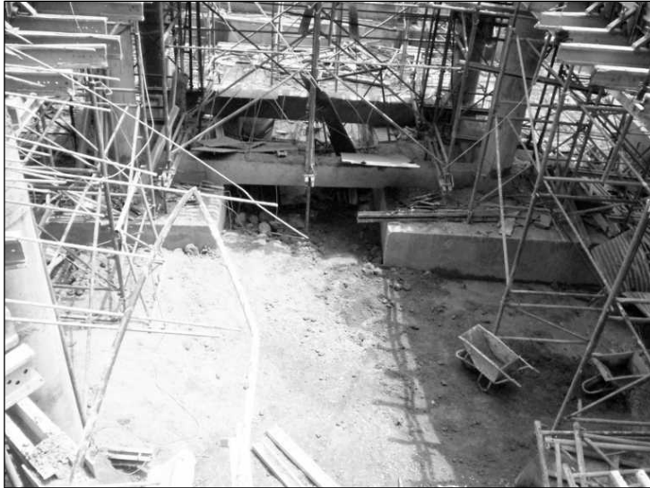
Figure 17.11 View of Portion of Slab and Beam Formwork which Collapsed.
