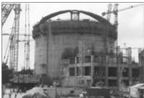
Figure 8.6 Erection of Dome Formwork.
