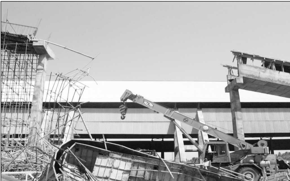
Figure 17.5 Collapse of Deck Slab between the Two Piers.
