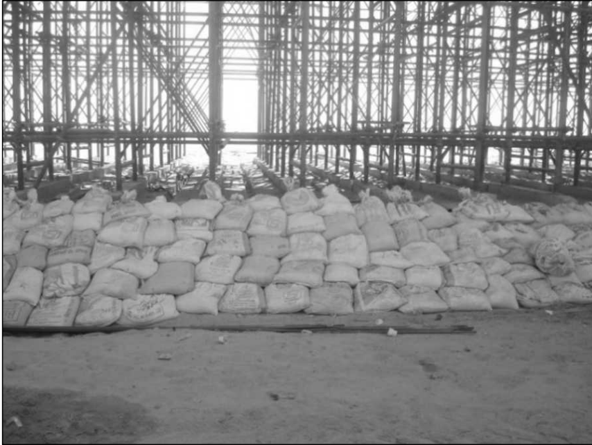
Figure 9.24 Arrangement of Sand Bags to Prevent Erosion of Soil Underneath the Scaffold.
