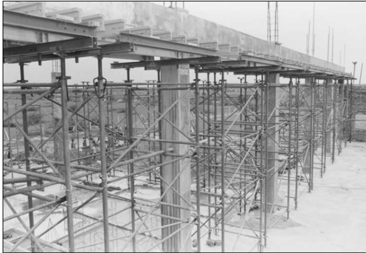
Figure 7.15 A Heavy Duty Tower in Position for Beam Formwork.
