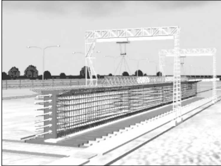
Figure 14.29 Casting Arrangement at the Precast Yard.
