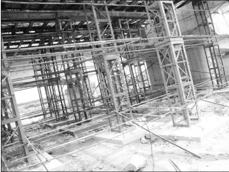
Figure 17.31 Reinforcement Bars Tied with Binding Wire Used as Horizontal Bracing.
