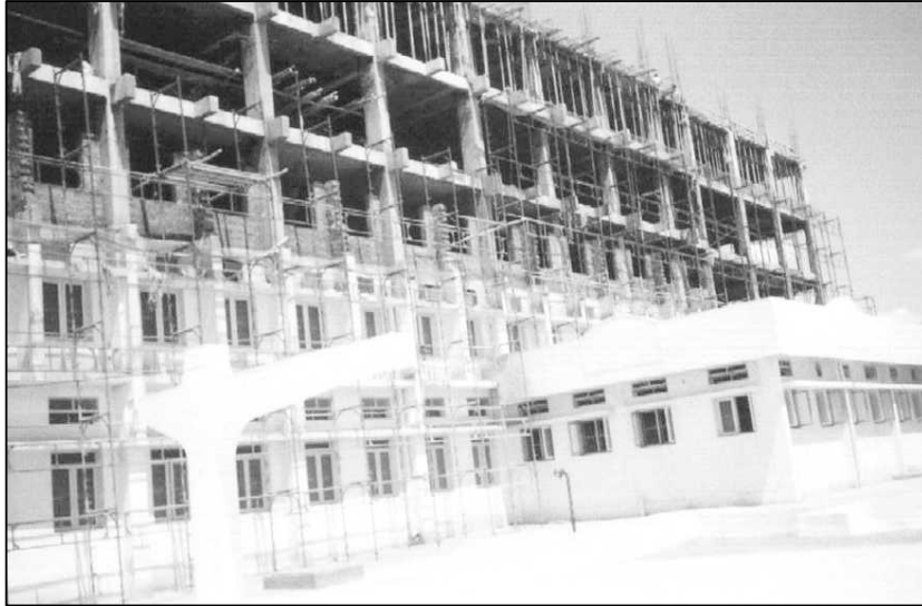
Figure 13.14 L&T Access Scaffold in Use for an Under Construction Building.
