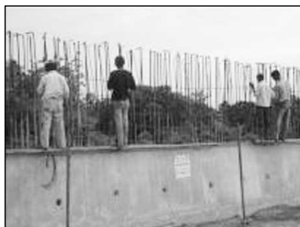
Figure 17.37 No PPEs. No Platform. No Access/Approach. No Display of Caution Signs.
