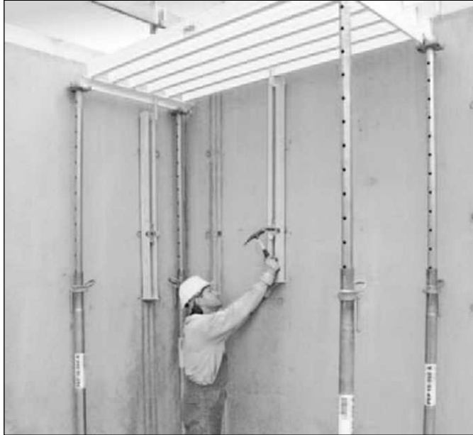
Figure 7.21 Wall Supports Being Installed for Both the Longitudinal and Transverse Directions (Courtesy PERI).
