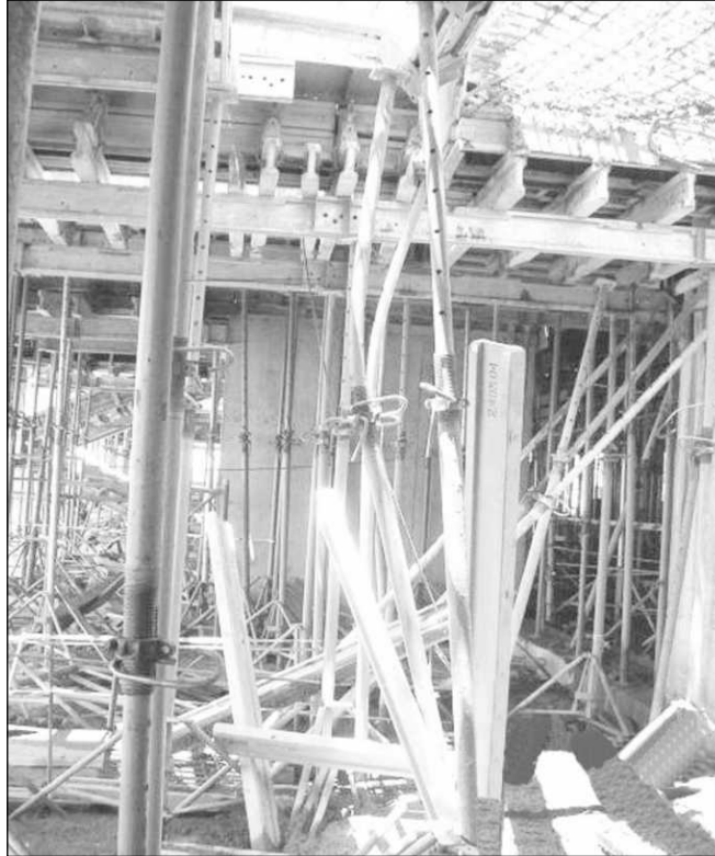
Figure 17.8 View of the Portion of the Slab which Failed due to Concrete Overloading.
