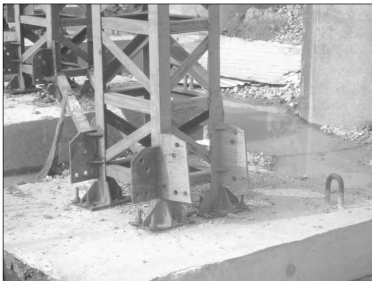
Figure 9.32 Connection Details of Trestle with Concrete Pedestal.
