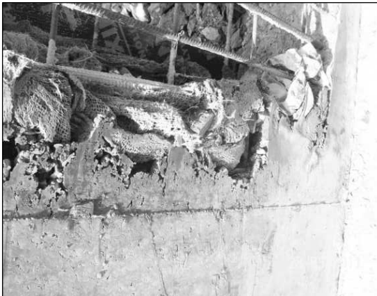
(c) Poor Construction Joint
