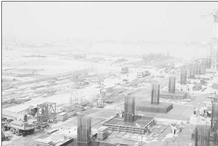
Figure 4.7 Large Column Footing at Delhi International Airport.
