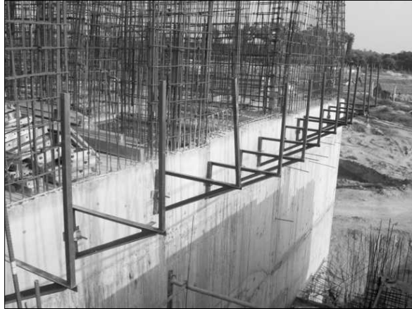
Figure 7.43 Erection of Brackets for the Upper Floor.
