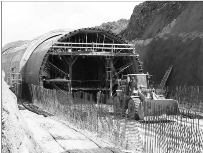
Figure 8.28 Cut and Cover Construction Method in Use for Tunnel Construction (Courtesy Doka).
