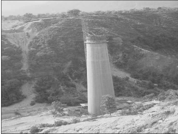
Figure 9.14 Construction of Pier Using Climbing Form (Jammu Udhampur Rail Link Project).
