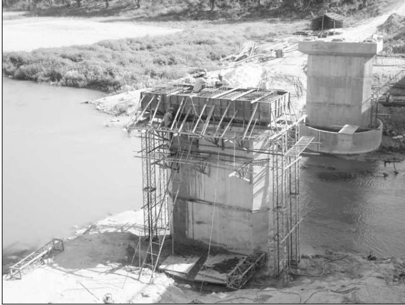
Figure 17.40 No Provision of Handrails and Lifeline Support.
