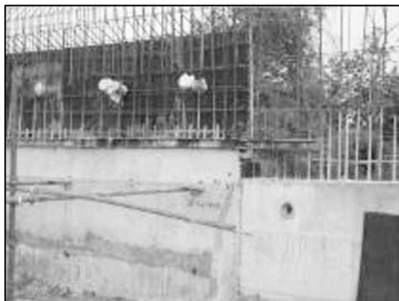
Figure 17.36 Scaffolding Pipes Are Erected on the Weepholes Made in the RCC.
