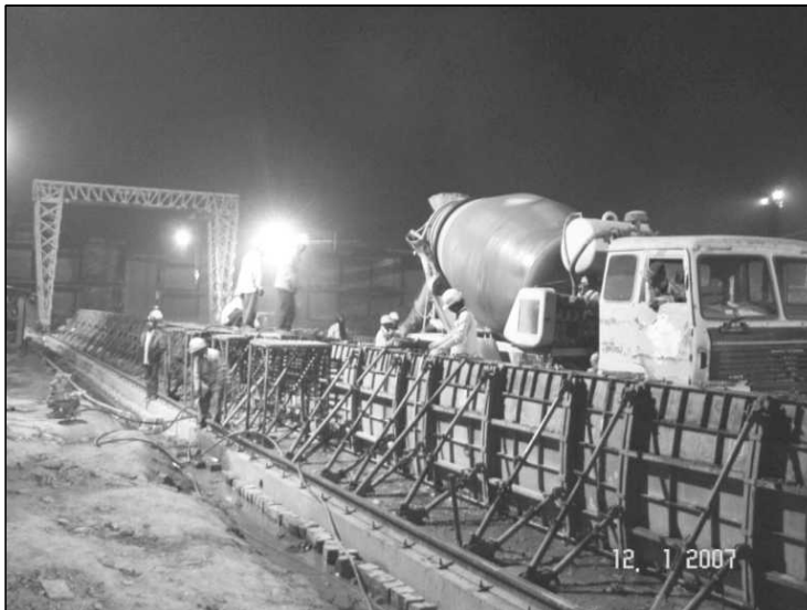
Figure 14.36 Casting Arrangement of Precast Crash Barrier.
