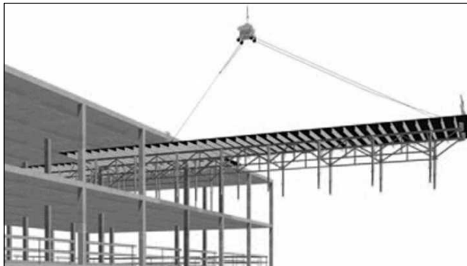
Figure 10.23 Skytable Form (See the Trusses) (Courtesy PERI).
