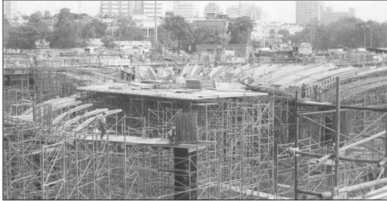
Figure 8.12 View Showing Shoring Towers Supporting the Dome Formwork Under Progress.
