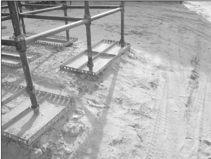
Figure 17.30 Shuttering Plates Being Used as Pedestal (Even Worse, They Are Kept on Loose Soil).
