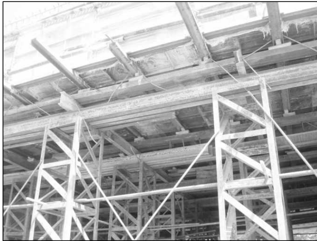
Figure 12.18 Typical Arrangements of Trestles.
