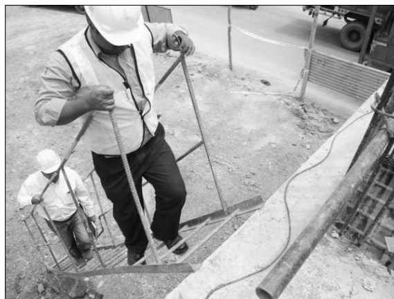
Figure 17.21 Makeshift Ladder of Inadequate Height and Unsafe.
