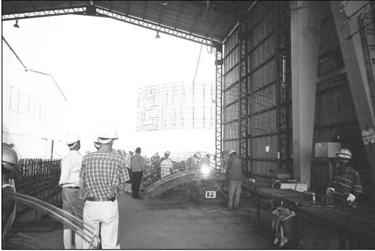
Figure 14.35 Pre-fabricated Reinforcement Cage for the Tunnel Element Being Lifted.
