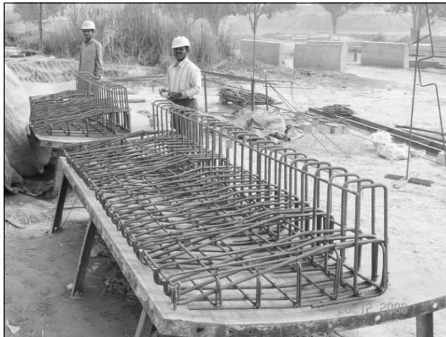
Figure 14.38 Prefabricated Reinforcement Cages Ready for Placement in the Crash Barrier Mould.
