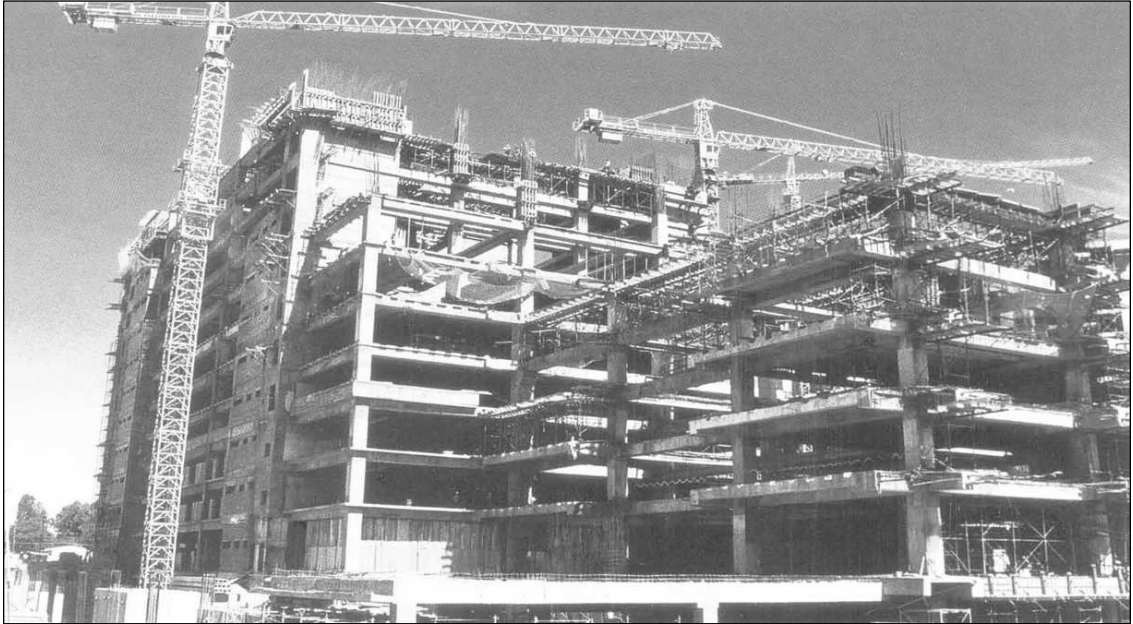
Figure 1.5 Proprietary Formwork for Casting Varied Concrete Elements Such As Wall, Column, and Slab and Beam Formwork (Courtesy L&T Formwork)
