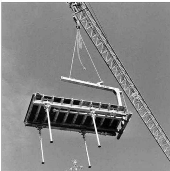
Figure 10.20 Table Module Being Transported Using Crane (Note the Lifting Fork) (Courtesy PERI).
