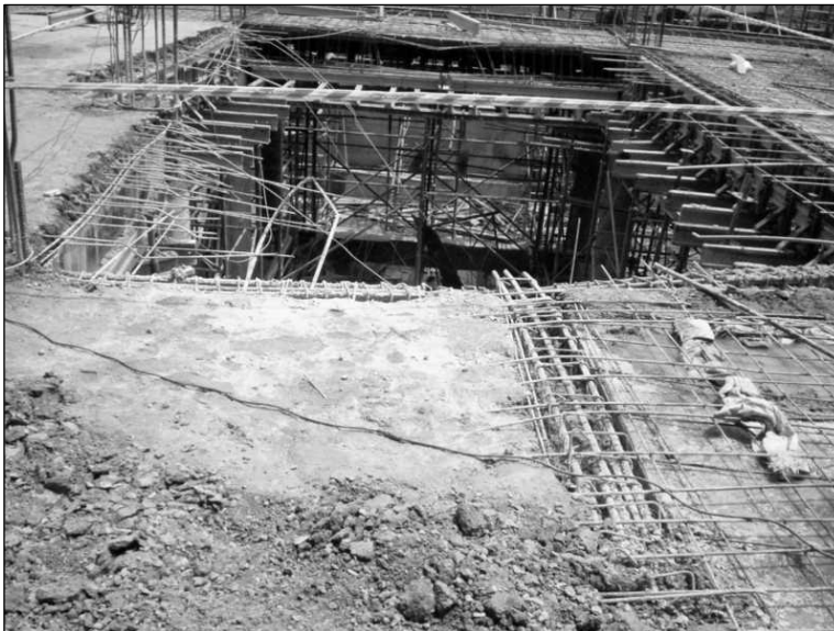
Figure 17.12 Another View of Portion of Slab and Beam Formwork which Collapsed.
