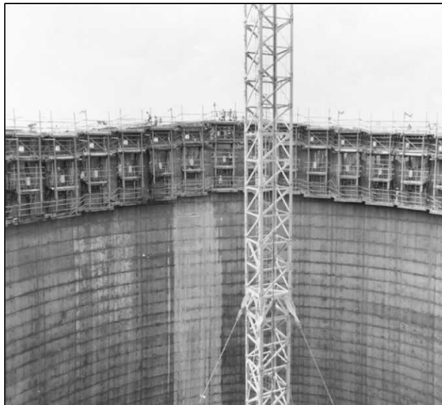
Figure 8.22 Inside View of the Natural Draft Cooling Tower Being Constructed Using Cooling-Tower Formwork.
