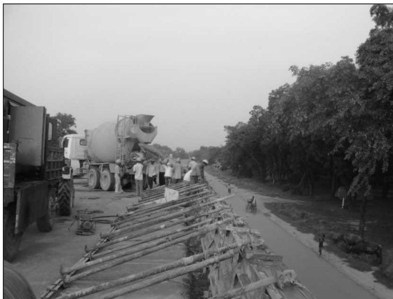
Figure 9.41 Formwork Arrangement of Parapets for a Typical Flyover/Bridge Project.
