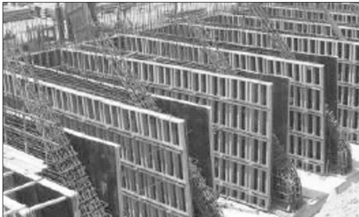
Figure 5.12 Field Application of L&T Wall Formwork System.
