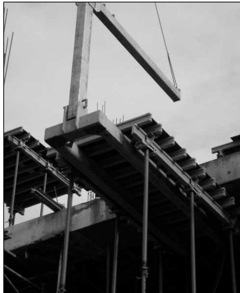
Figure 10.14 Table Formwork Being Flown to its New Location (Courtesy L&T Formwork).
