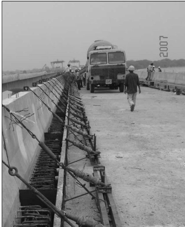
Figure 9.43 Temporary Support for Precast Parapet.
