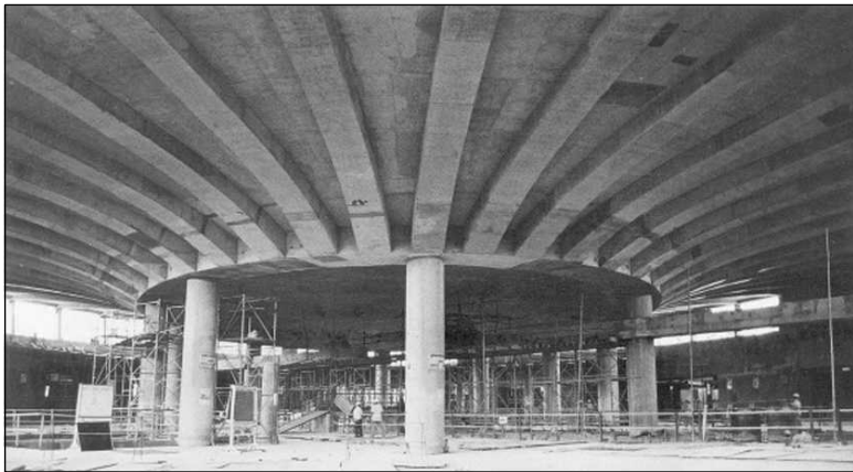
Figure 8.13 Completed View of the Dome Shell.
