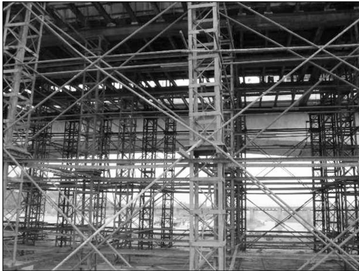
Figure 17.32 Reinforcement Bars Tied With Binding Wires Being Used as Diagonal Bracings.
