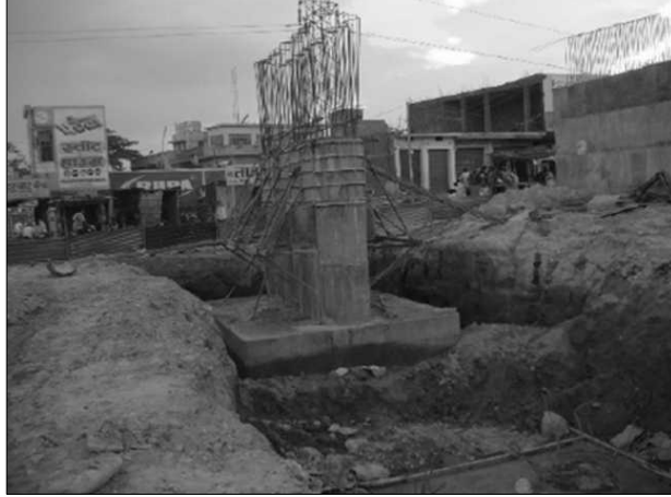
Figure 9.8 Round Pier Under Construction (LMNHP-Package 12).
