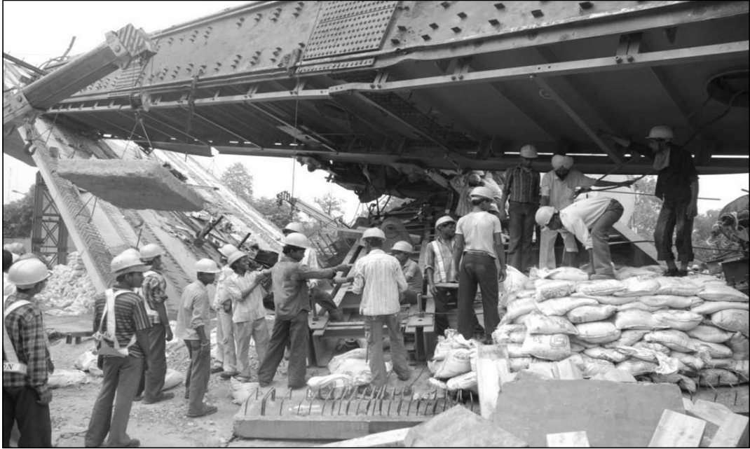
Figure 9.48 View of Zamrudpur Under Construction Metro Bridge Span Collapse.
