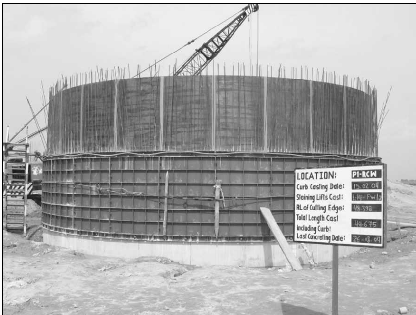
Figure 9.6 View of Inside Shutter in Position for Next Lift.
