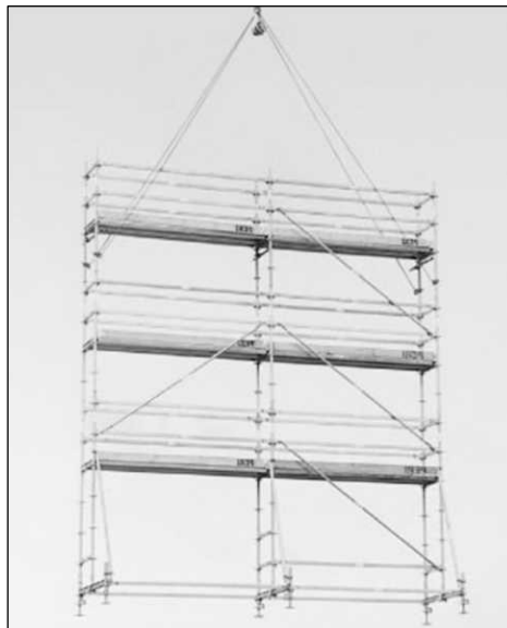
Figure 13.16 PERI UP Scaffold Being Shifted Using Crane (Courtesy PERI).
