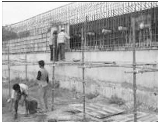
Figure 17.15 Formwork and Reinforcement Crew without Appropriate PPE.
