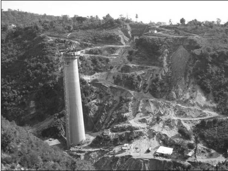
Figure 9.16 Construction of Pier Using Slipform (Jammu Udhampur Raillink Project).
