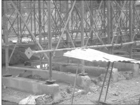
Figure 17.33 Foot Plates not in Proper Contact with Concrete Pedestals.
