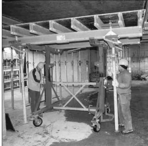
Figure 10.21 Table Form Being Shifted on Trolley to the Desired Location (Courtesy PERI).
