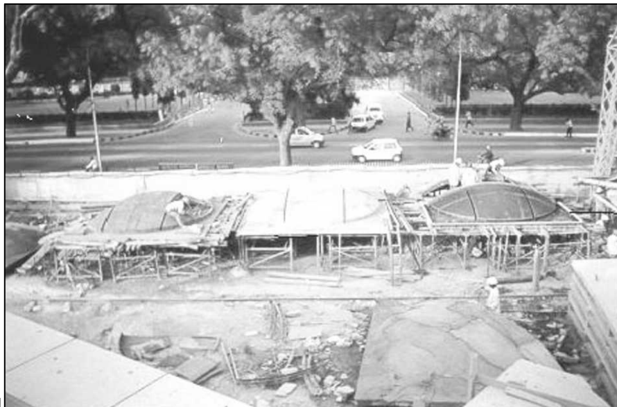
Figure 14.25 Casting of Bubbles in Progress for the Parliament Library Project.
