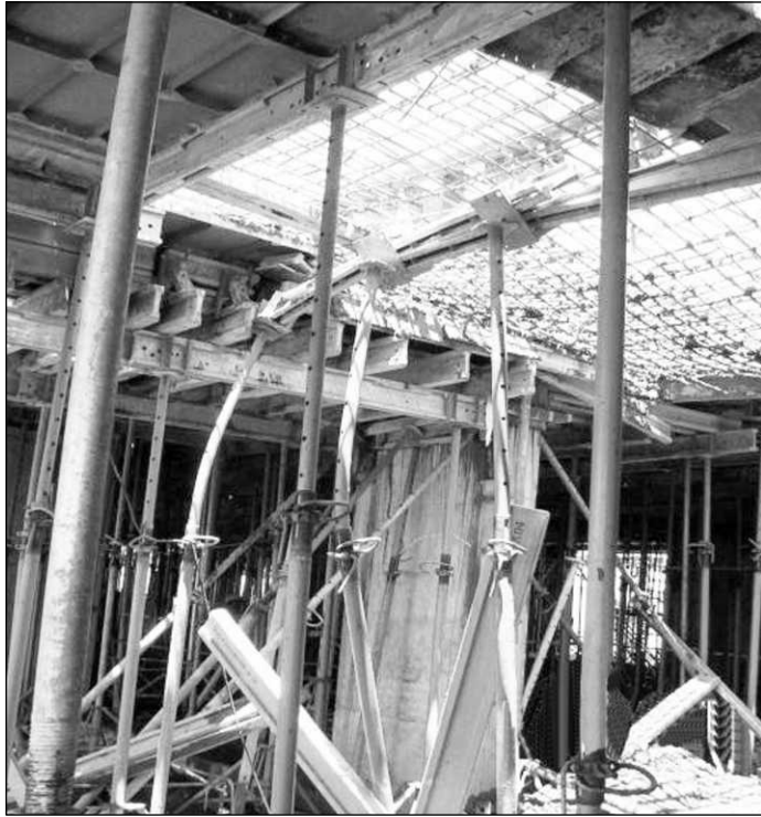
Figure 17.9 Another View of the Portion of the Slab which Failed due to Concrete Overloading (Note the Buckled Props).
