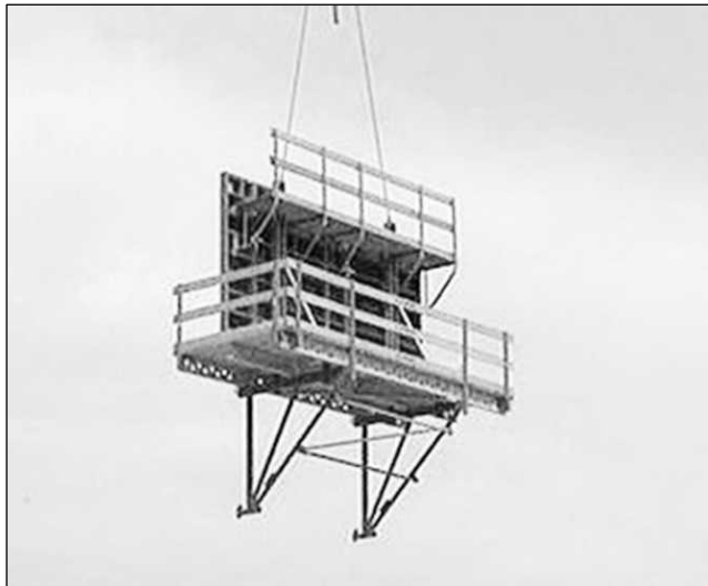
Figure 5.28 CB System Being Transported Through Crane (Courtesy PERI).
