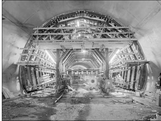
Figure 8.31 Mining Method of Construction in Use for a Tunnel Jobsite (Courtesy Doka).
