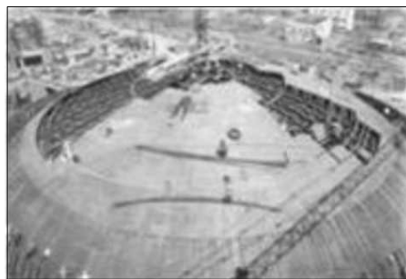
Figure 8.7 Dome Formwork Fixing.
