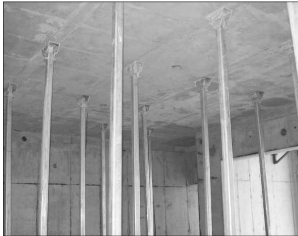
Figure 7.44 Left out Props in Position.
