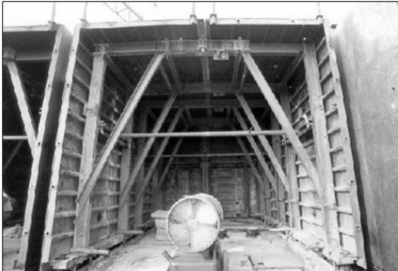
Figure 10.30 Heating Equipment in Position for the Tunnel Formwork.
