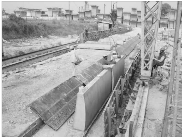
Figure 14.39 Demoulding in Progress for Crash Barrier.
