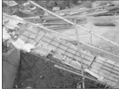
Figure 17.27 Access Ramps Made out of Shuttering Plates.
