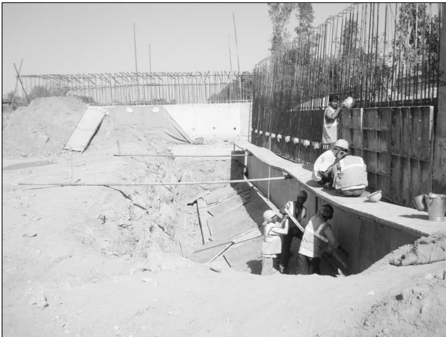
Figure 17.39 Workers on the Unstable and Weak Working Platform.
