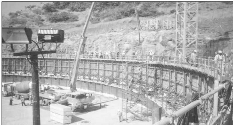
Figure 5.36 View of CB-150F in Use For Construction of an LNG Tank (Courtesy L&T Formwork).
