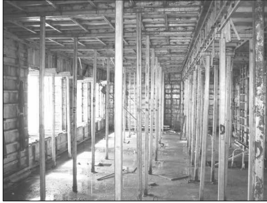
Figure 7.37 Deck Erection.
