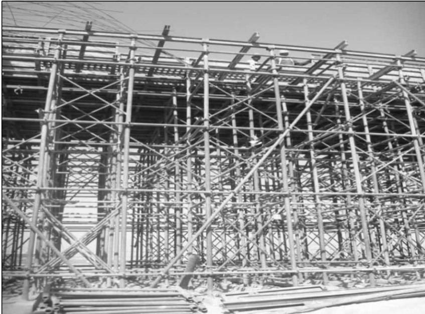
Figure 9.25 Tubular Steel Scaffold in Position (Note the Bracings).
