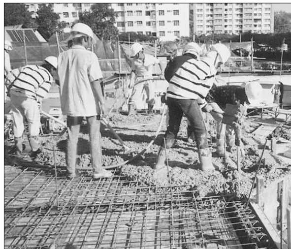
Figure 7.40 Concrete Pouring in Progress.
