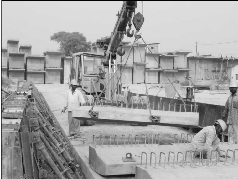
Figure 14.37 Handling Arrangement for Precast Crash Barrier.
