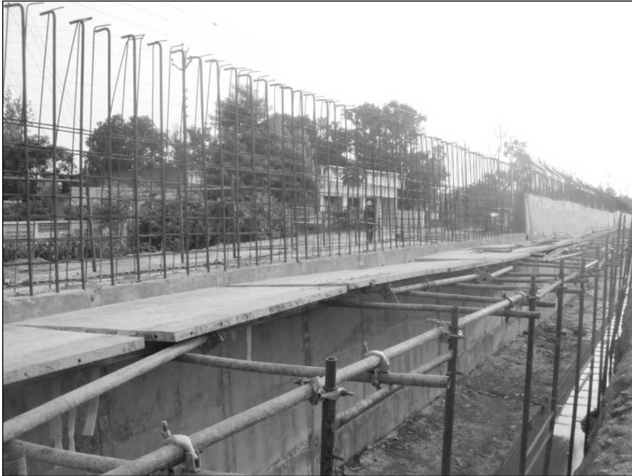
Figure 17.38 Improper Working Platform, No Hand Rails, No Foot Guards.
