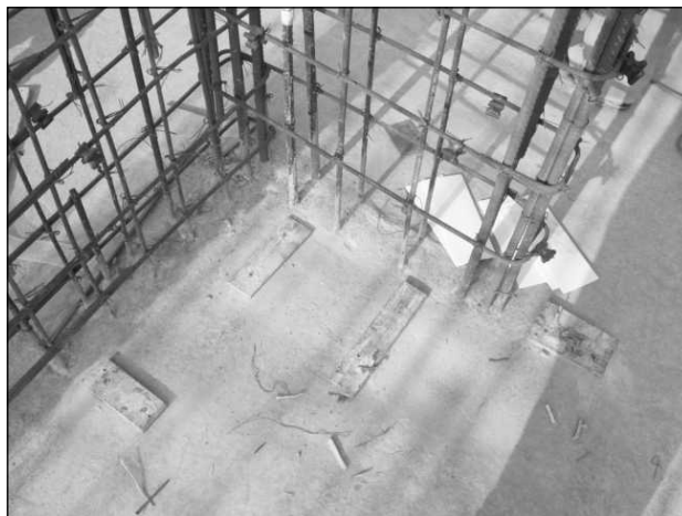
Figure 7.30 Setting Out and Timber Stay Fixing.
