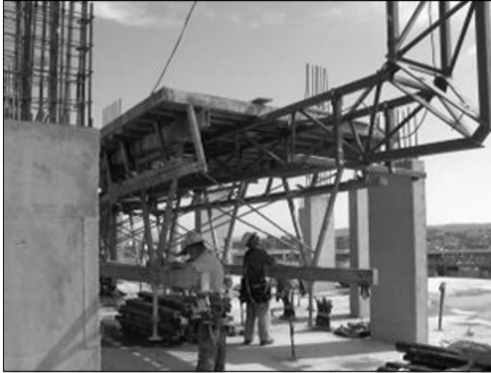
Figure 10.9 Positioning a Flying Form Table.
