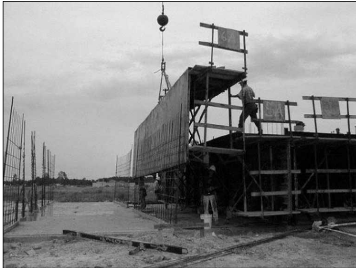
Figure 10.28 Placement of Tunnel Form in Progress.
