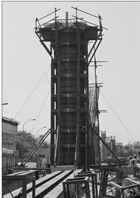
Figure 9.9 Formwork for Pier (Note: Casting in Single Pour).
