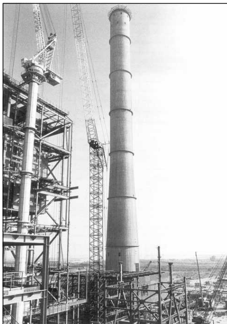
Figure 11.21 275 m High RCC Slipformed Tapered Chimney at 2 \times 500 MW Anpara Thermal Power Station in U.P.
