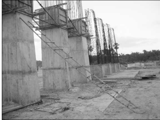
Figure 17.22 Ladder not Properly Rested.
