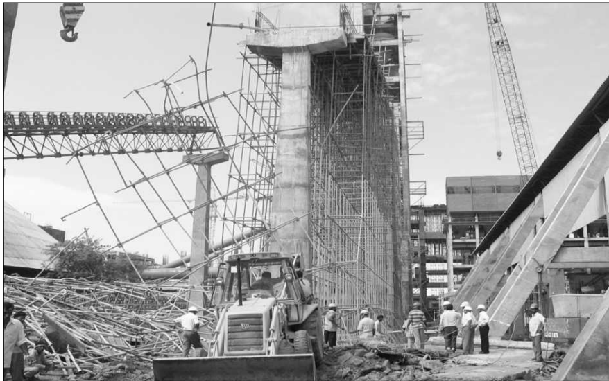
Figure 17.7 Shoring Tower in Position for the Deck Slab Adjacent to the Collapsed Slab.
