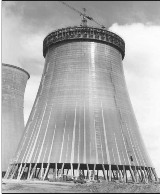
Figure 8.21 Natural Draft Cooling Tower Construction.
