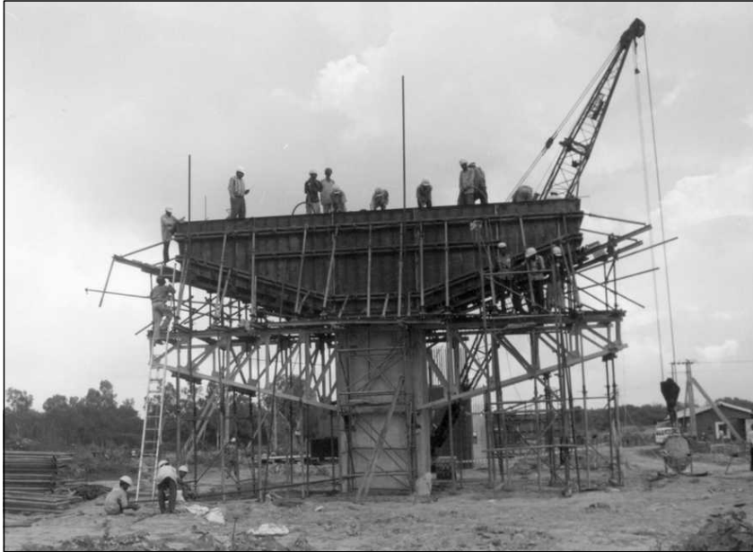
Figure 9.22 Formwork Arrangement for Pier Cap Used in the Construction of Flyover at Delhi.
