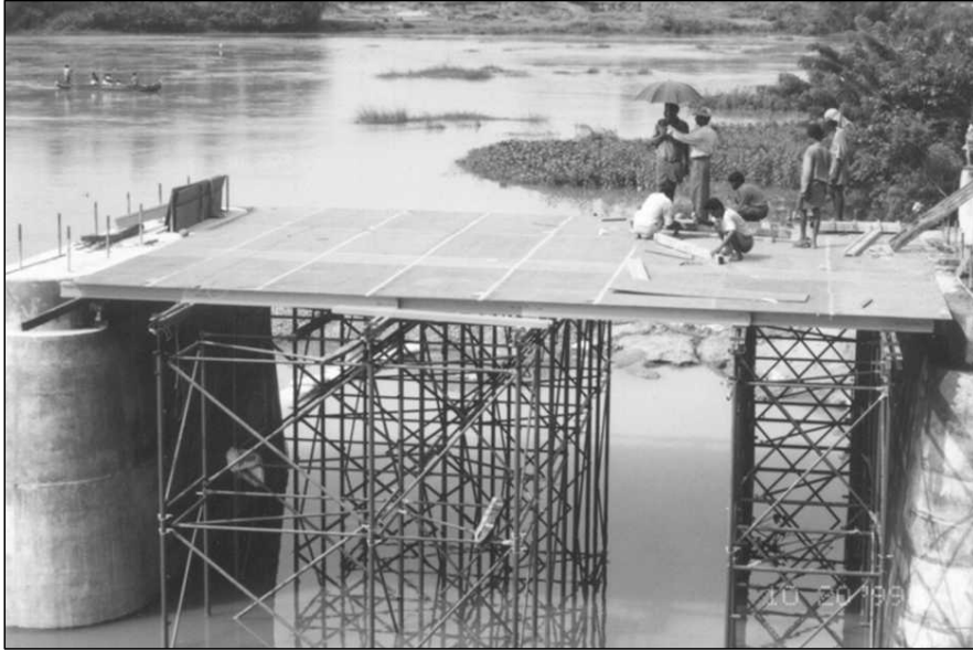
Figure 9.23 Formwork and Supporting Arrangement for Bridge Deck Slab Using Proprietary Formwork.
