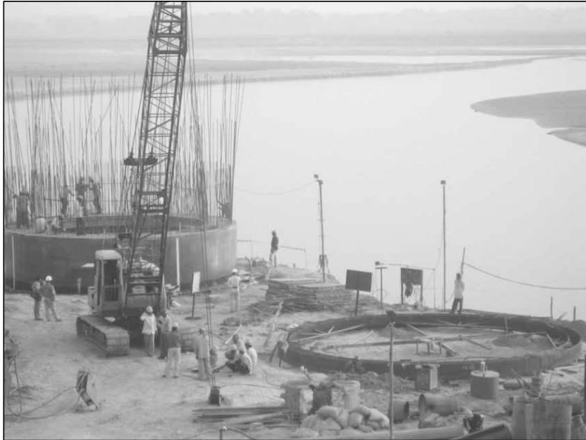
Figure 9.5 Reinforcement Tying for Next Lift in Progress for One Well and Cutting Edge Work in Progress in Other Well.
