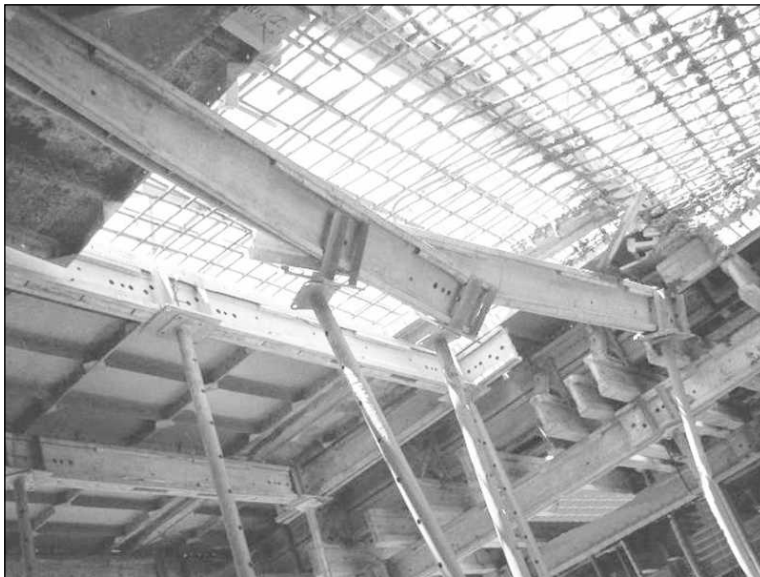
Figure 17.10 Another View of the Portion of the Slab which Failed due to Concrete Overloading.
