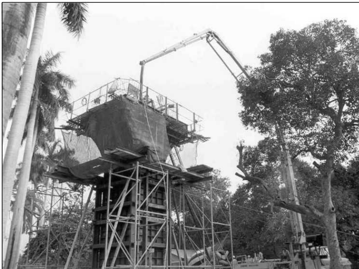
Figure 9.17 Formwork Arrangement for Pier and Pier Cap for Delhi Metro Project.
