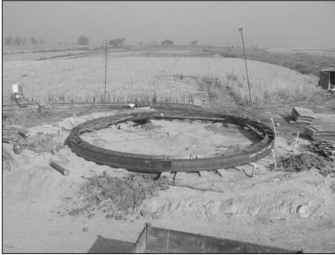
Figure 9.2 Cutting Edge of a Caisson for a Circular Well.
