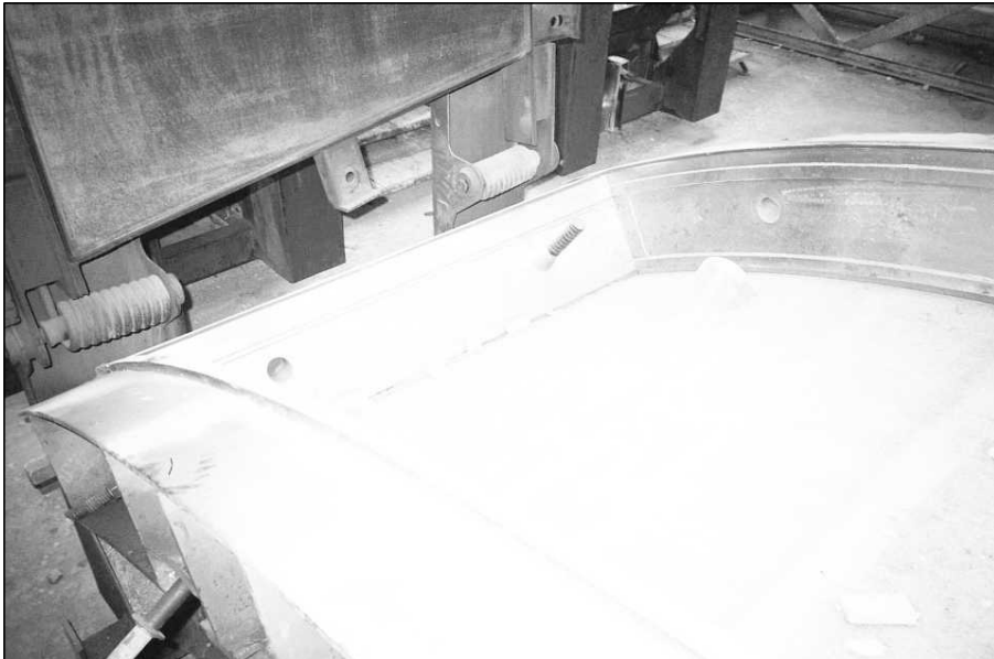
Figure 14.34 Mould for Tunnel Element in Position.
