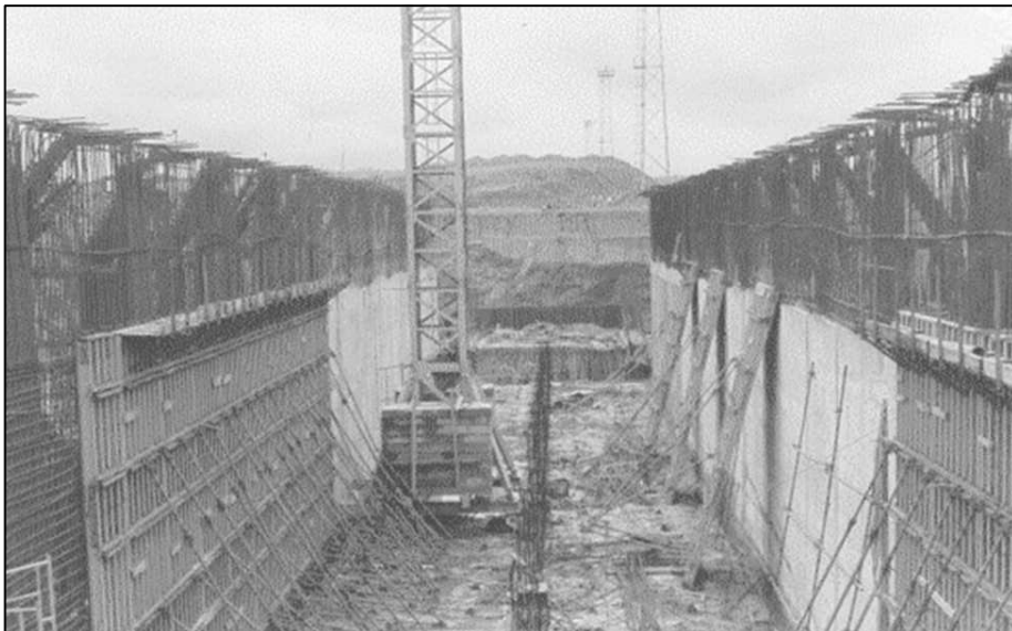
Figure 10.34 Construction of Track Hopper at Anpara Super Thermal Power Station Project Executed by L&T- ECC Construction Group.
