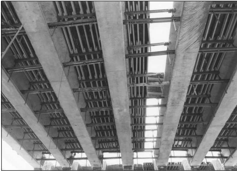
Figure 9.40 Formwork Arrangement for Deck Slab.
