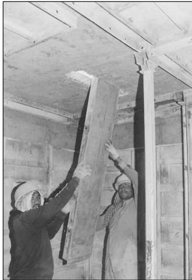
Figure 7.42 Lifting through Openings.
