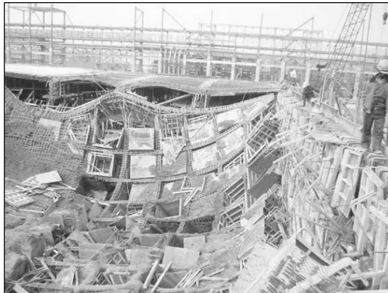
Figure 17.3 Another View of Collapsed Waffle Slab Segment.
