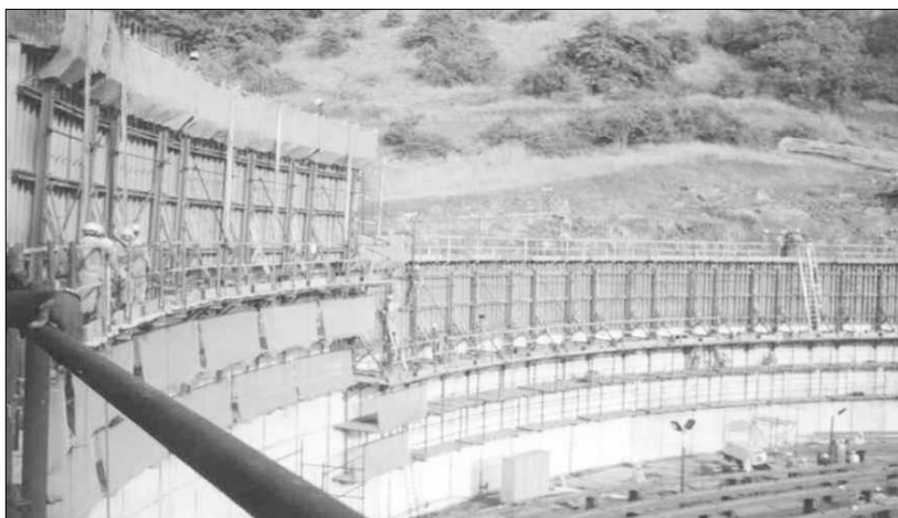
Figure 5.37 Another View of CB-150F in Use For Construction of an LNG Tank (Courtesy L&T Formwork).
