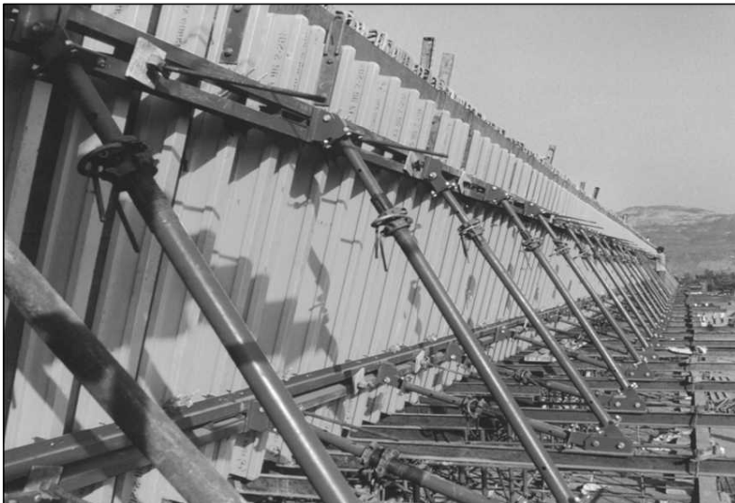
Figure 9.29 Closer View of Form Arrangement for Web of Box Girder.
