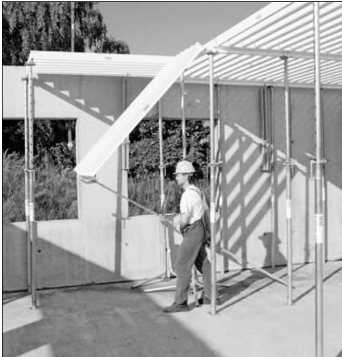
Figure 7.22 Gridflex Panels Being Erected from the Existing Floor (Courtesy PERI).
