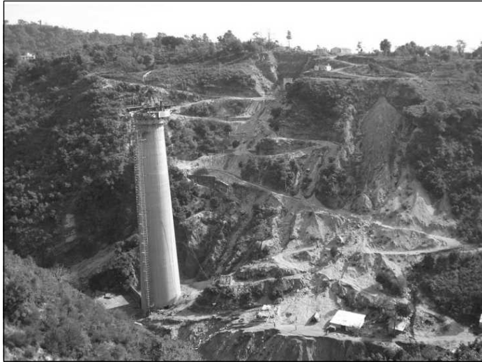
Figure 11.22 Construction of Pier (Jammu Udhampur Raillink Project).
