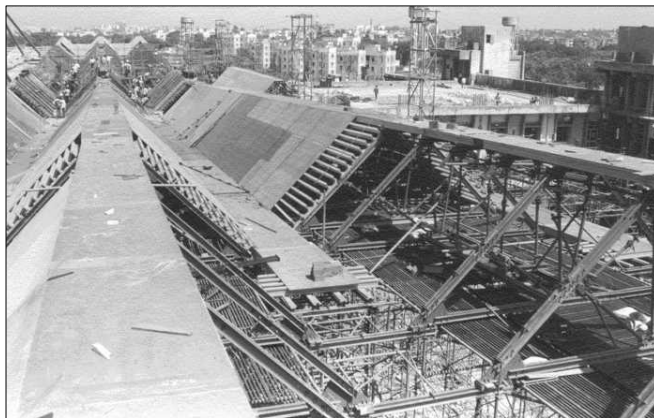
Figure 8.15 Formwork Using Standard Components of L&T Formwork Systems to Form the Folded Plate Slab of Air Hangar at Mumbai.
