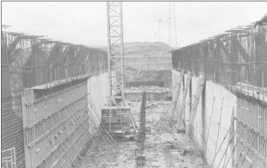
Figure 5.2 Application of Large Area Wall Formwork in Track Hopper Construction.
