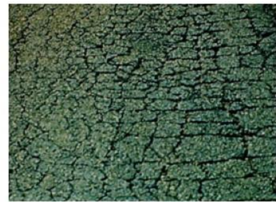
Fatigue cracking –interconnected cracks
