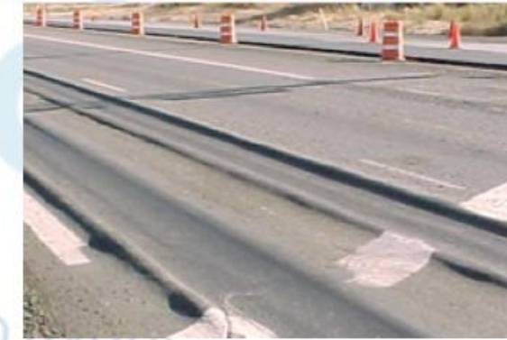
Surface depression in the wheel path.
