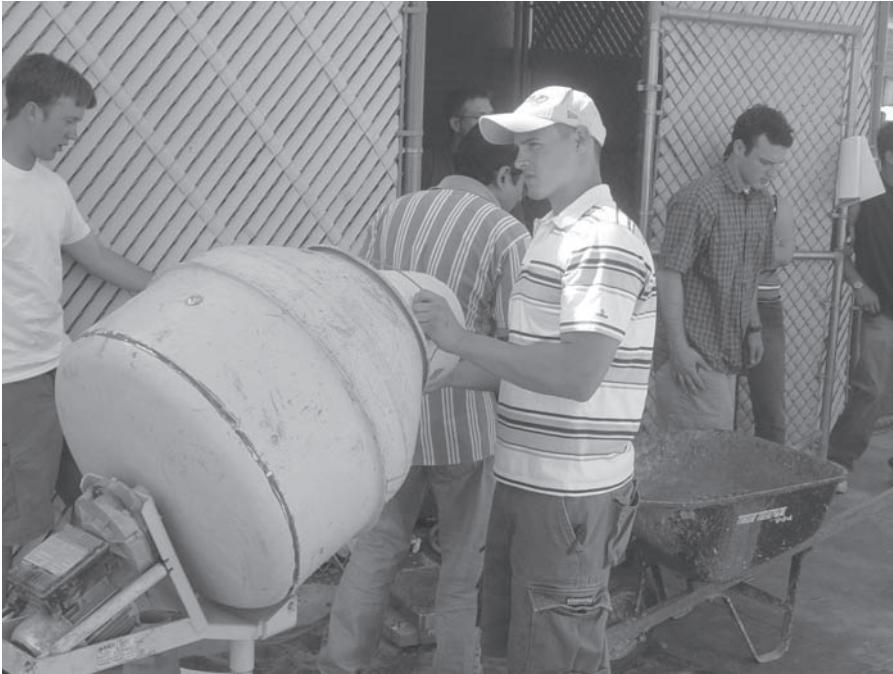
FIGURE A.30 Mixing concrete in a mixer.
