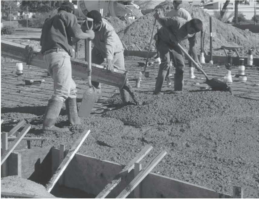
FIGURE 7.8 Placing concrete slab.
