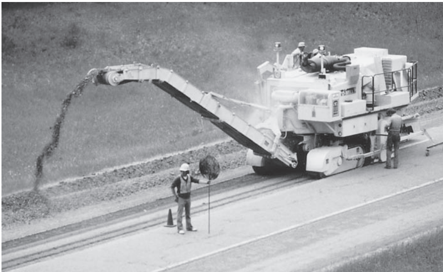
FIGURE 9.41 Milling old pavement.
