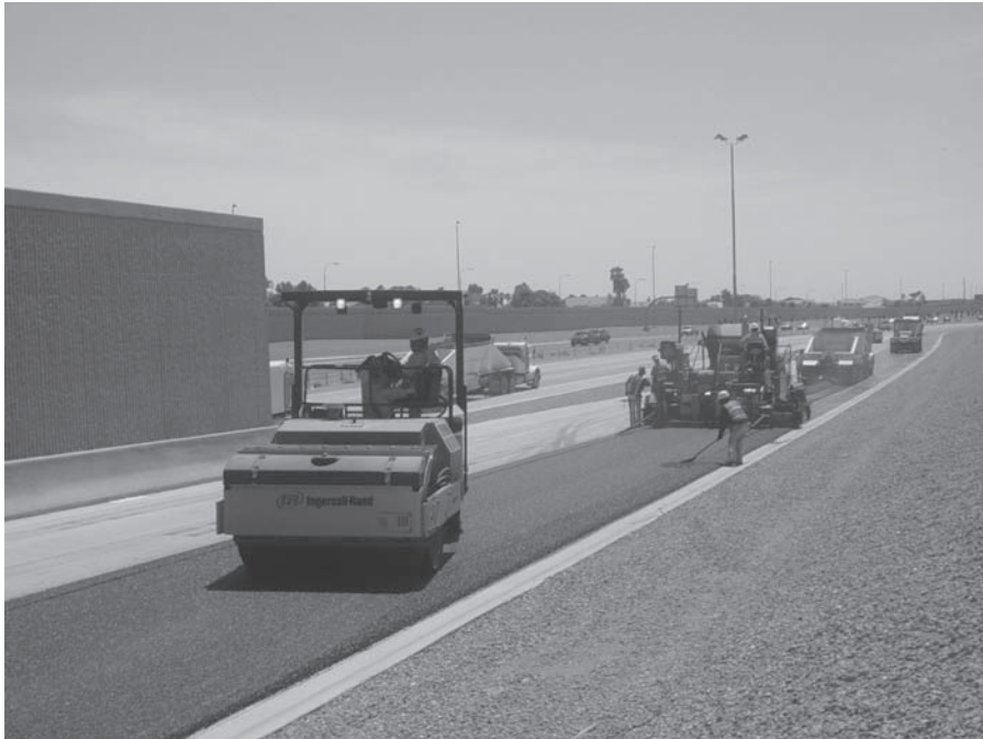
FIGURE 9.6 Compaction of asphalt concrete.
