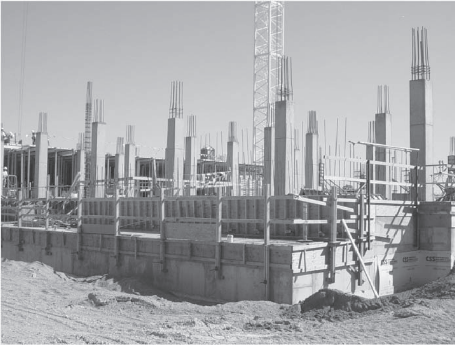
FIGURE 3.13 Steel rebars used to reinforce PCC columns.
