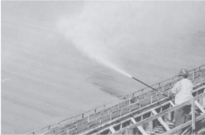
FIGURE 7.26 Curing concrete by fogging. (Courtesy of FHWA)
