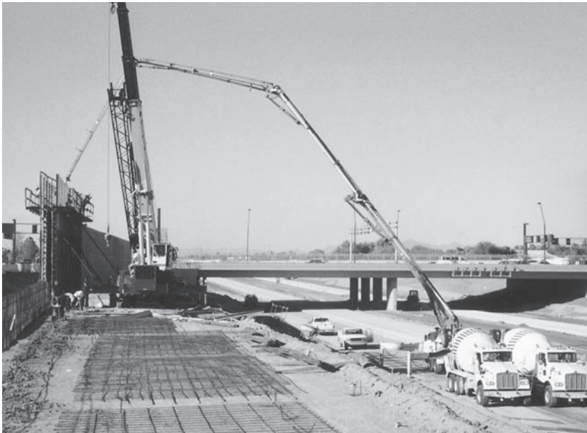
FIGURE 7.12 Pumping concrete in a retaining wall.
