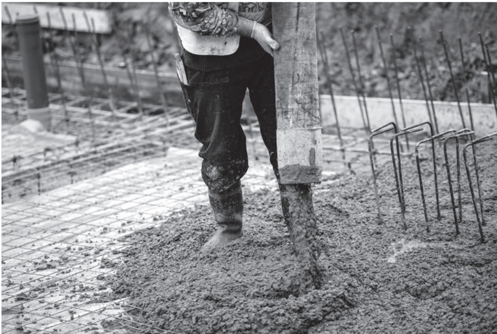
FIGURE 7.9 Placing concrete with Chute. (Fotolia/Hoda Bogdan)
