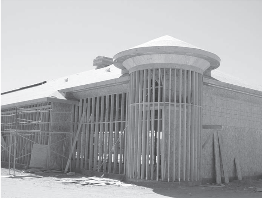
FIGURE 10.1 Wood frame used for building structural support.
