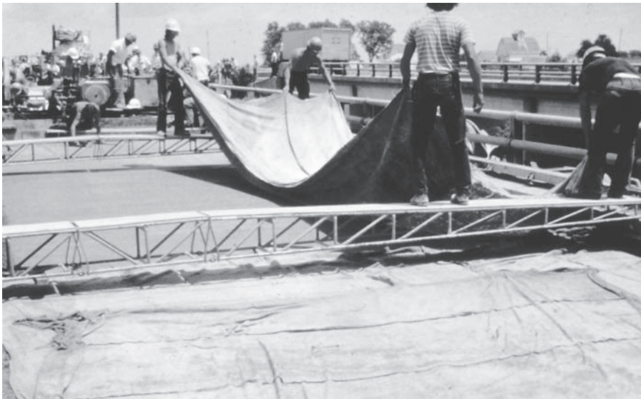
FIGURE 7.28 Curing concrete with impervious fabrics.
