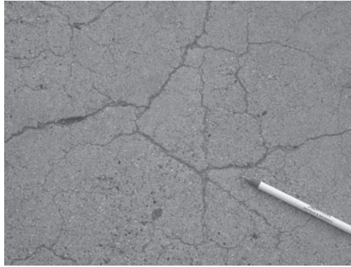
FIGURE 5.19 Example of cracking in concrete due to alkali–silica reactivity.
