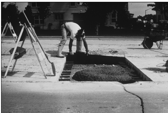
Figure 21.3 Full-depth repair with dowels and fiberboard for isolation. (From American Concrete Pavement Association (ACPA). 1996a. Construction of Portland Cement Concrete Pavements, Participant's Manual , FHWA HI-96-027, AASHTO/FHWA/INDUSTRY Joint Training, Washington, D.C.: Federal Highway Administration, United States Department of Transportation. Available on the web at http://isddc.dot.gov/OLPFiles/FHWA/014737.pdf : VIII-41.)
