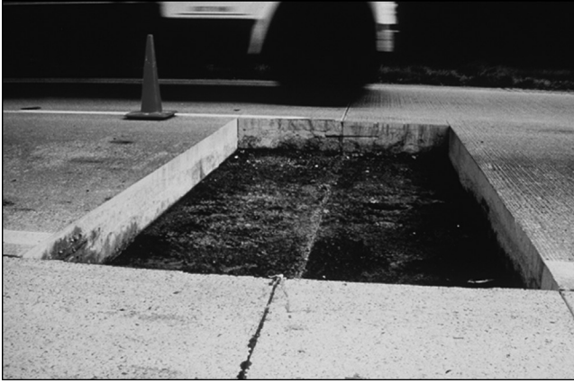
Figure 21.1 Hole prepared for a full-depth repair at a joint. (From American Concrete Pavement Association (ACPA). 1996a. Construction of Portland Cement Concrete Pavements, Participant's Manual, FHWA HI-96-027 , AASHTO/FHWA/INDUSTRY Joint Training, Washington, D.C.: Federal Highway Administration, United States Department of Transportation. Available on the web at http://isddc.dot.gov/OLPFiles/FHWA/014737.pdf : VIII-28.)
