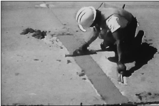
Figure 21.2 Partial-depth repair. (From American Concrete Pavement Association (ACPA). 1996a. Construction of Portland Cement Concrete Pavements, Participant's Manual, FHWA HI-96-027 , AASHTO/FHWA/INDUSTRY Joint Training, Washington, D.C.: Federal Highway Administration, United States Department of Transportation. Available on the web at http://isddc.dot.gov/OLPFiles/FHWA/014737.pdf : VIII-57.)
