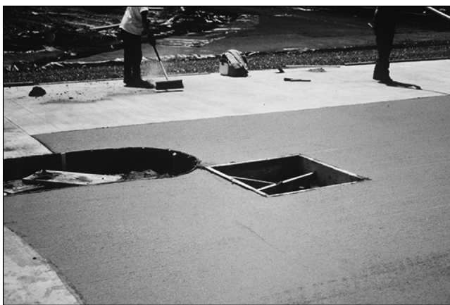
Figure 18.11 Blockouts for utility, drainage, and similar structures. (Adapted from American Concrete Pavement Association (ACPA). 1996a. Construction of Portland Cement Concrete Pavements, Participant's Manual, FHWA HI-96-027 , AASHTO/FHWA/INDUSTRY Joint Training, Washington, D.C.: Federal Highway Administration, United States Department of Transportation. Available on the web at http://isddc.dot.gov/OLPFiles/FHWA/014737.pdf : VI-91.)
