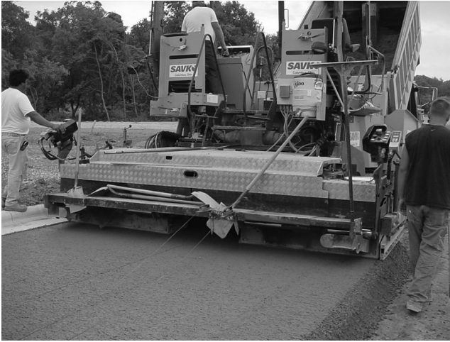
Figure 2.10 RCC pavement construction—Columbus, Ohio. (Photo by author.)
