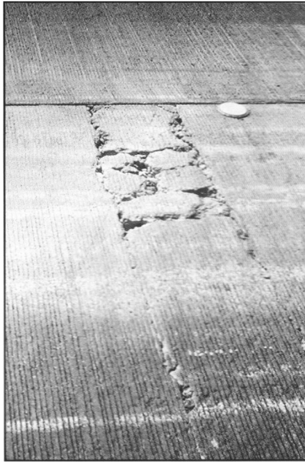
Figure 4.12 High severity punchout. (From Miller, J.S. and Bellinger, W.Y. 2003. Distress Identification Manual for the Long-Term Pavement Performance Program (Fourth Revised Edition) , FHWA-RD-03-031, p. 79. Washington, DC: Federal Highway Administration, United States Department of Transportation.)
