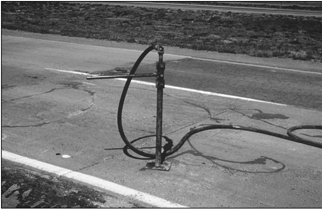
Figure 21.6 Grout injection for slab stabilization. (From American Concrete Pavement Association (ACPA). 1996a. Construction of Portland Cement Concrete Pavements, Participant's Manual , FHWA HI-96-027, AASHTO/FHWA/INDUSTRY Joint Training, Washington, D.C.: Federal Highway Administration, United States Department of Transportation. Available on the web at http://isddc.dot.gov/OLPFiles/FHWA/014737.pdf : VIII-23.)
