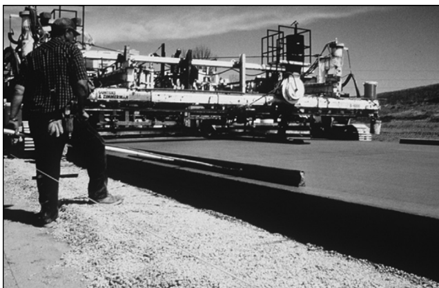
Figure 18.2 Concrete pavement produced by slipforming. (Adapted from American Concrete Pavement Association (ACPA). 1996a. Construction of Portland Cement Concrete Pavements, Participant's Manual , FHWA HI-96-027, AASHTO/FHWA/INDUSTRY Joint Training, Washington, D.C.: Federal Highway Administration, United States Department of Transportation. Available on the web at http://isddc.dot.gov/OLPFiles/FHWA/014737.pdf : VI-6.)
