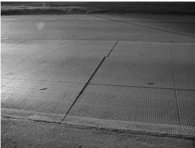
Figure 22.9 Failure of UTW by panel sliding. (Photo by the author).
