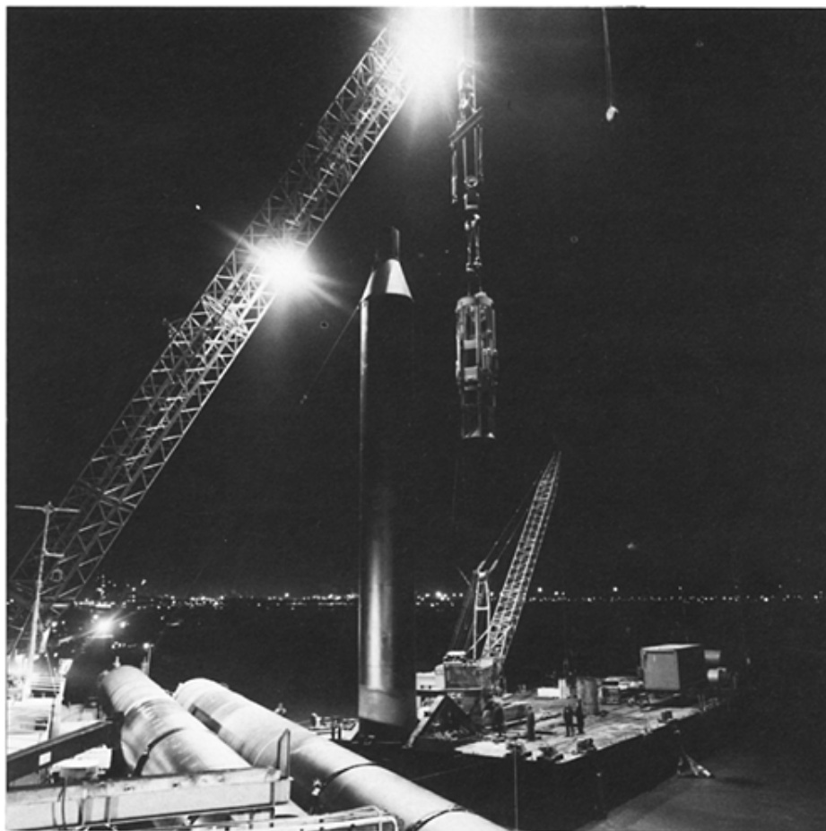
Fig. 3.15 BSP International Foundations Ltd. 40-tonne hydraulic hammer
