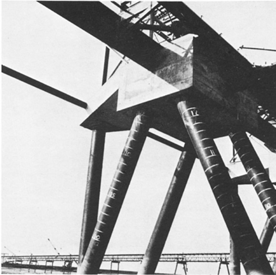
Fig. 8.2 Raking and vertical piles used to restrain berthing forces in bulk handling jetty
