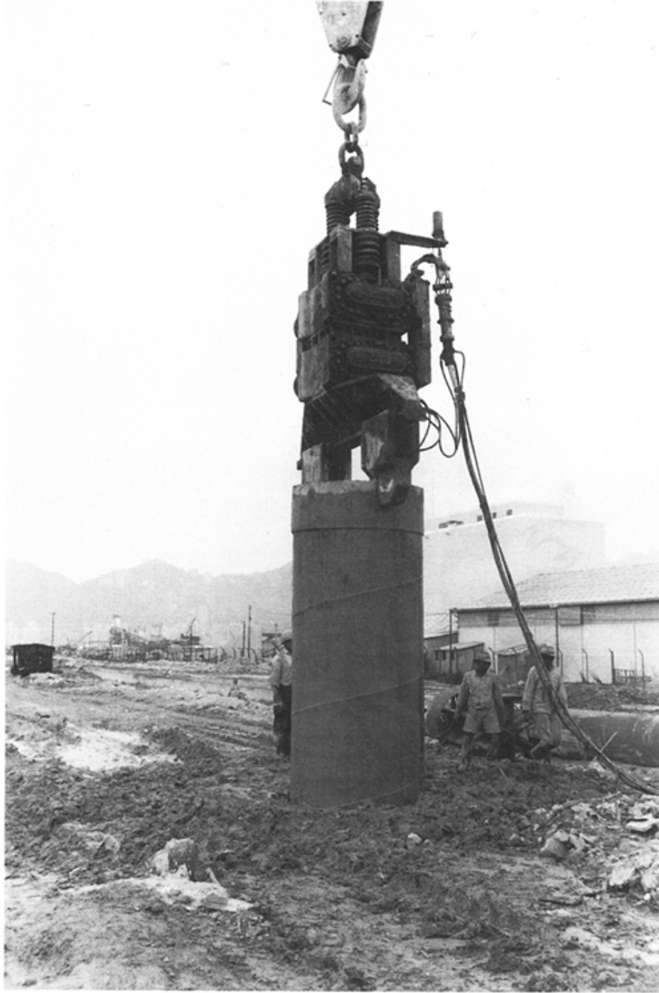
Fig. 3.17 Driving pile casing with Muller vibrator.
