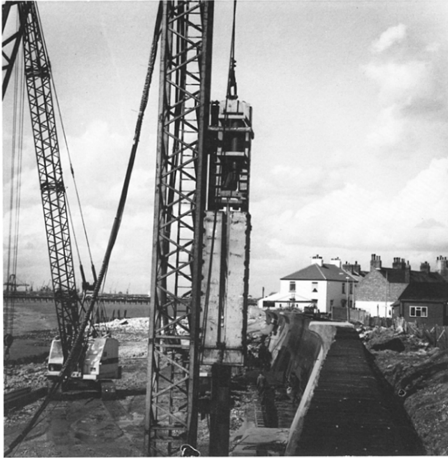
Fig. 3.14 BSP International Foundations Ltd. hydraulic piling hammer
